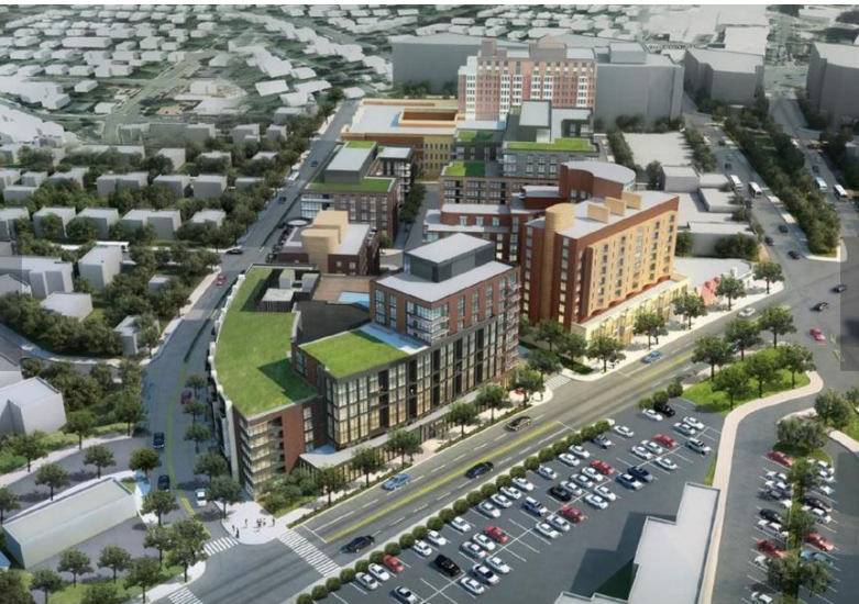
High land value taxes incentivize development of vacant or underutilized parcels. Example of a redeveloped parking lot in Arlington, VA above
