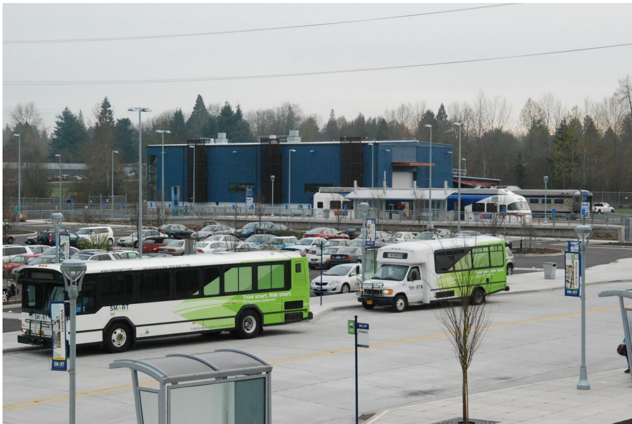
SMART bus routes and TriMet Westside Express (WES) commuter rail service meet at SMART Central at Wilsonville Station.
