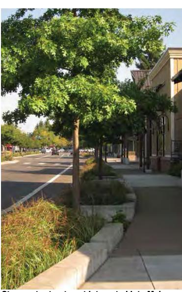
Stormwater treatment integrated into Main Street
