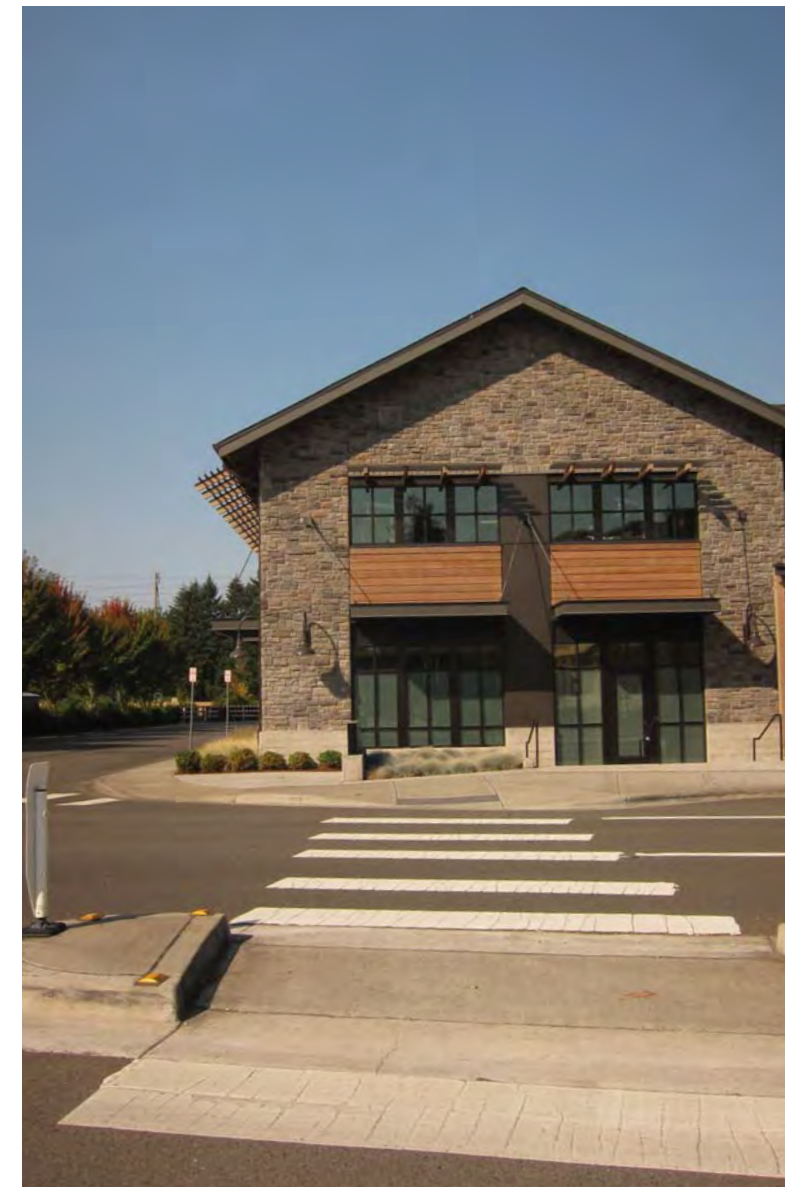
Zebra Crossing (Provides wide, visible and safe crossing)
