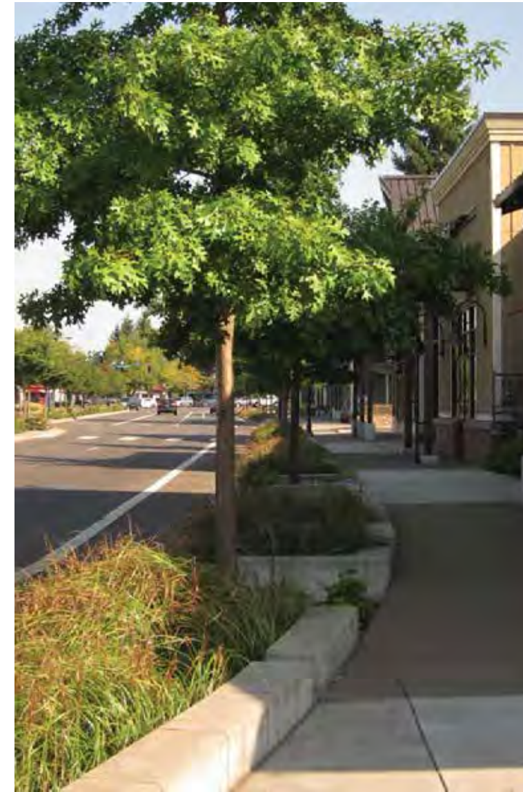
Stormwater treatment integrated into Main Street
