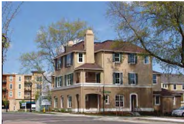
High-Density Residential (Small Condominium)
