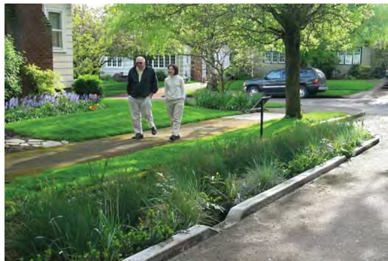
Stormwater Bioswale (Natural detention and filtration of on-street rainwater)
