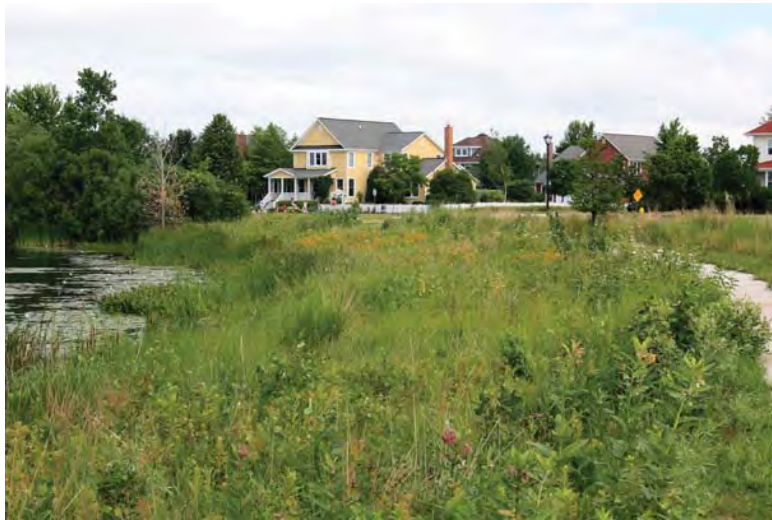
Retention Pond (Holds rainwater in wetland environment)
