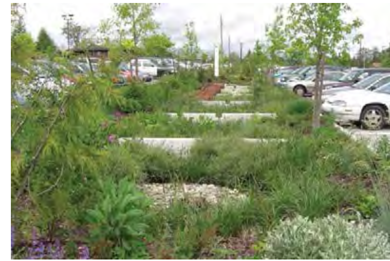
Parking Lot Rain Garden (Natural detention and filtration of parking lot rainwater)
