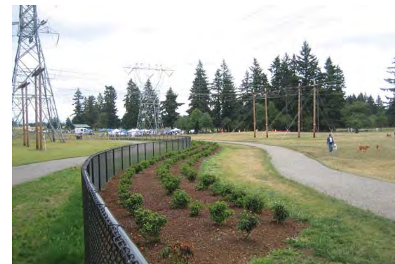
Park integrated with powerline easement
