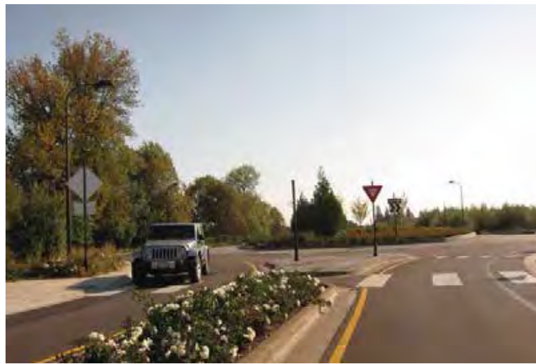
Pedestrian Refuge at Roundabout
