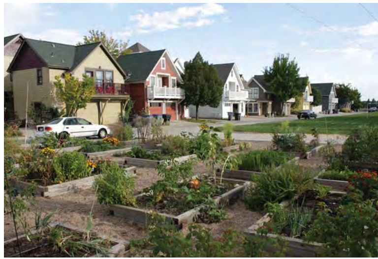
Homes overlooking community garden
