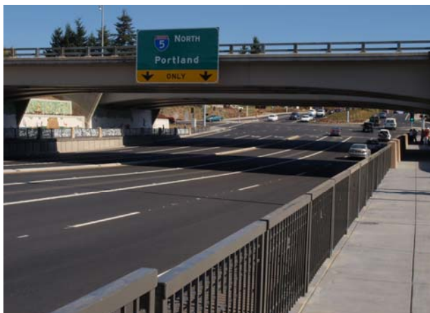
Looking east to the I-5/Wilsonville Road interchange. Interchange areas have the most restrictive access spacing standards to ensure safety and mobility.
