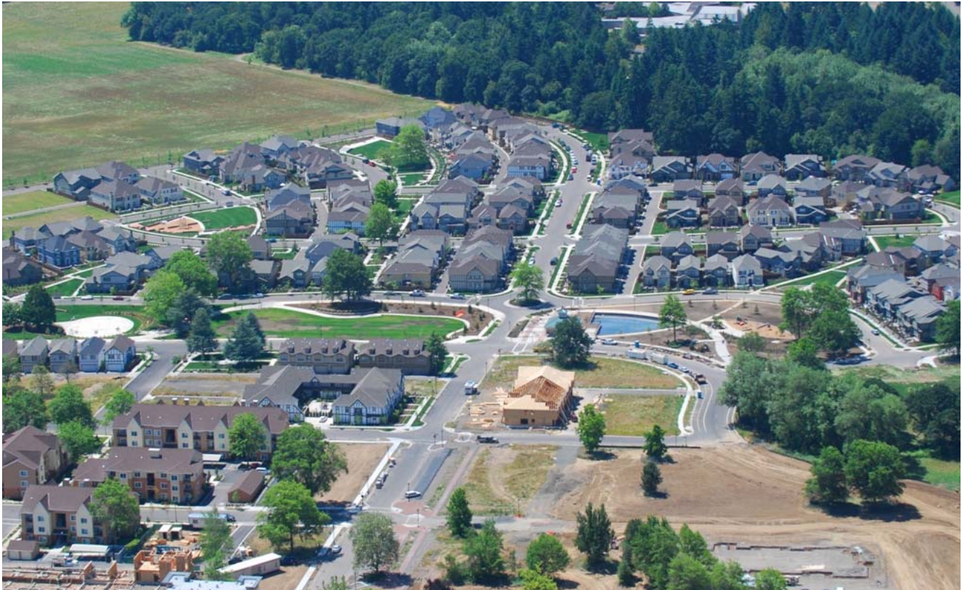
Villebois Village Master Plan was designed to provide a high level of connectivity for all travel modes using short blocks arranged in a grid pattern, numerous pathways, and a diversity of land use.
