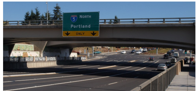
Looking east to the I-5/Wilsonville Road interchange.
