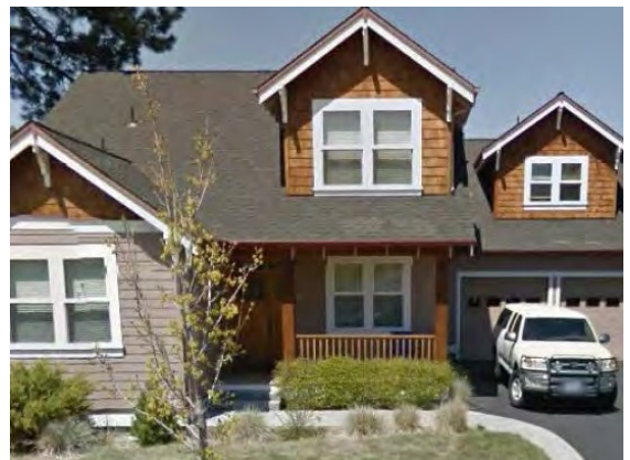
Recessed garages help to create a more attractive neighborhood street.
