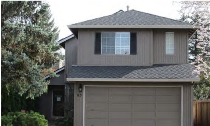
Houses where windows and doors are hidden from the street detract from the perceived safety of the neighborhood, because no one is aware of what happens in the street.
