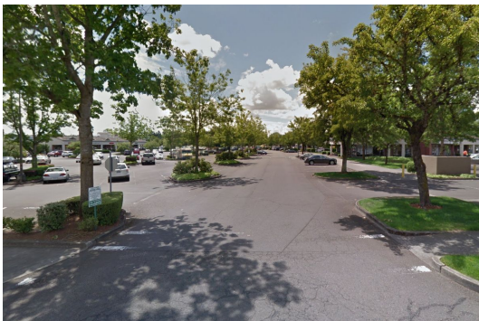
LOCATION IN.4 Potential new "Framework" street to extend Park Ave to Wilsonville Road
