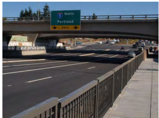
The Interstate-5/Wilsonville Road interchange serves as a key regional connection while also providing connectivity between east and west Wilsonville.
