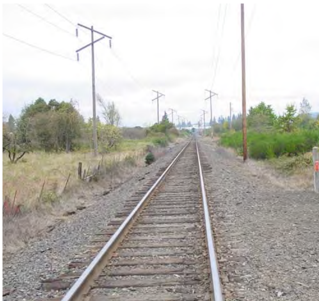
Portland and Western's Oregon Electric rail line runs north/south through Wilsonville and serves as an important freight and commuter rail corridor. However, it also creates a barrier to travel for other modes due to limited crossing locations.
