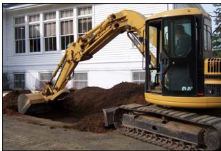
Figure 10A. Mix compost into the soil as deeply as possible. Add about \frac{1}{3} compost by volume. For large areas or areas with compacted soil, consider heavy equipment.
