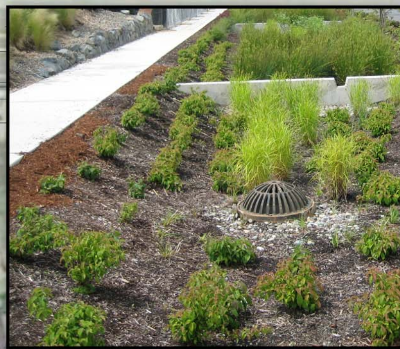
1 STORMWATER MANAGEMENT FACILITY
