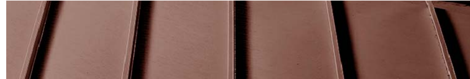
STANDING SEAM METAL ROOF
