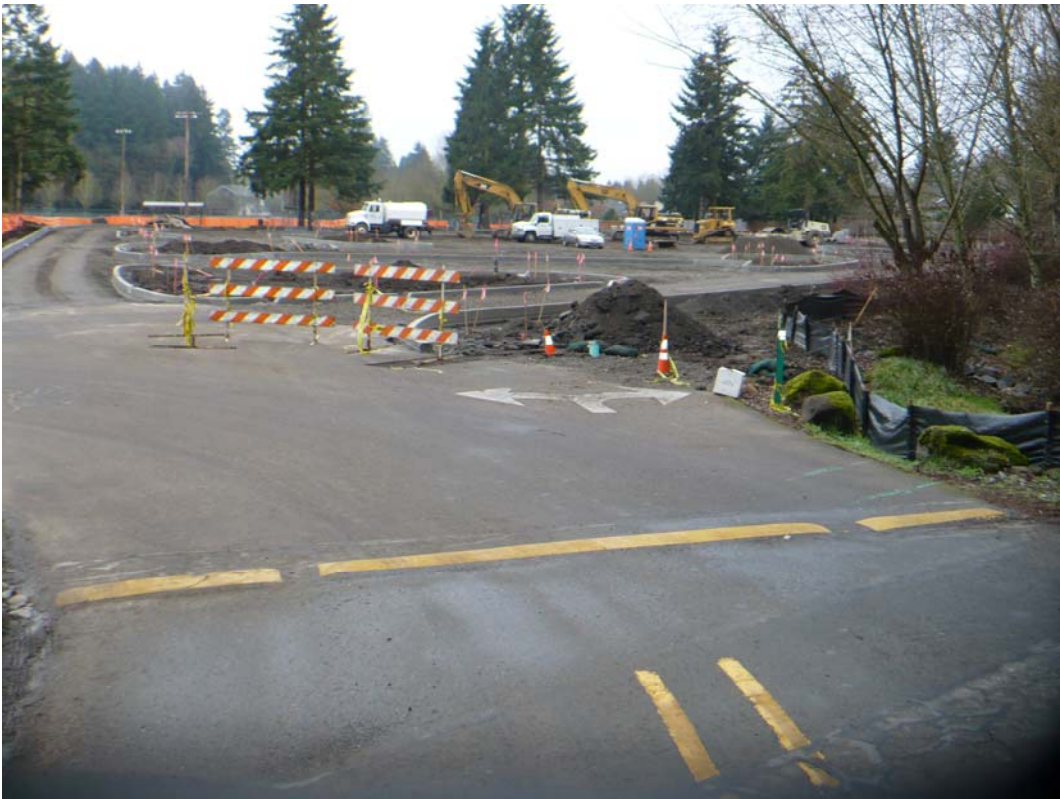
View looking south at perimeter drive aisle and new islands
