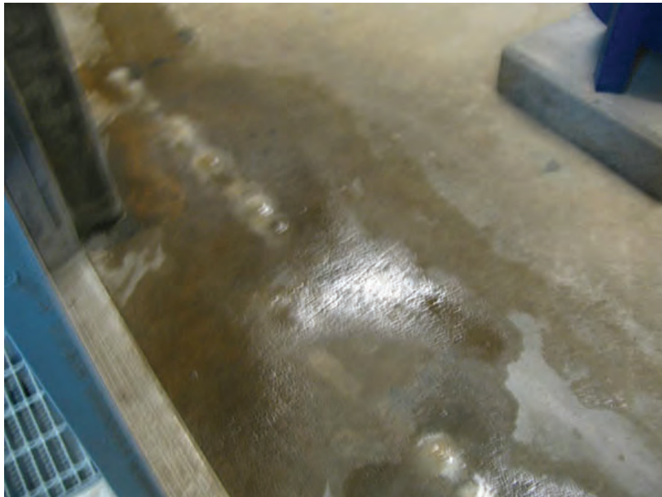
Photo 18 – LS9 – Water on the floor of the south blower room at the Filter Gallery due to active leaks from the water channels above.
