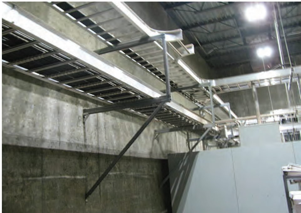
Photo 36 – S12 – The cable tray within the High Service PS lacks longitudinal seismic bracing.
