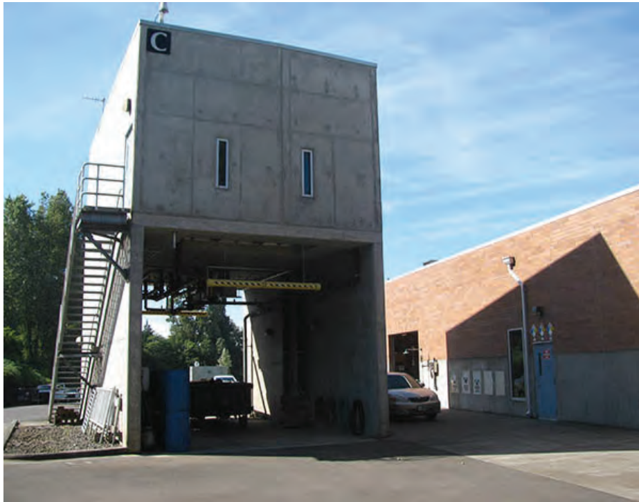
Photo 31 – S7 – The Solids Dewatering Building has no lateral load resisting system at the lower level in the east-west direction.
