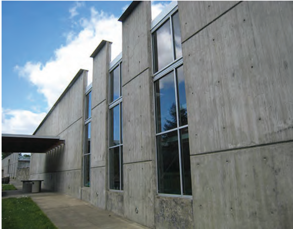
Photo 29 – S5 – Diaphragm chord splices at the windows along the west wall require strengthening.
