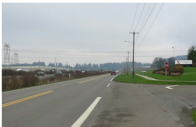
Parkway Avenue near the Xerox campus is a Minor Arterial but does not include bike lanes. There is a sidewalk on the east side, but it ends at the boundary with the vacant parcel to the north.
