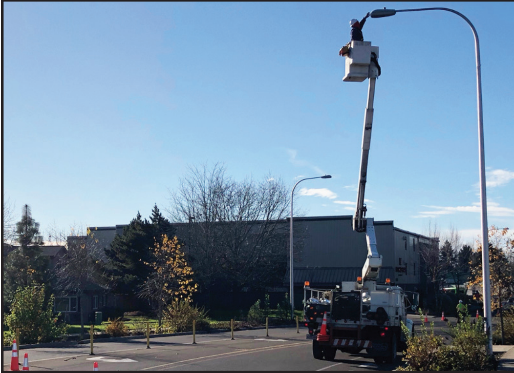
LED streetlight conversion project - light installation.
