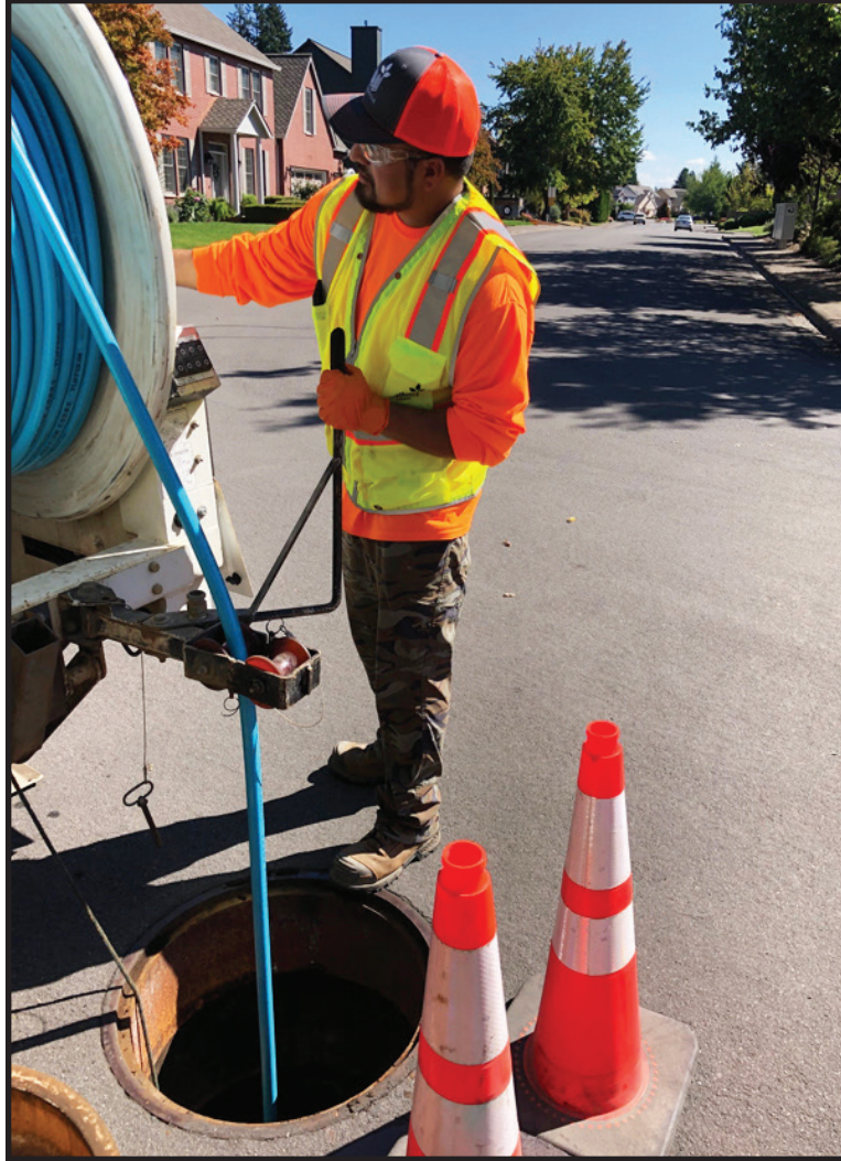
Staff cleaning wastewater pipes throughout the City.
