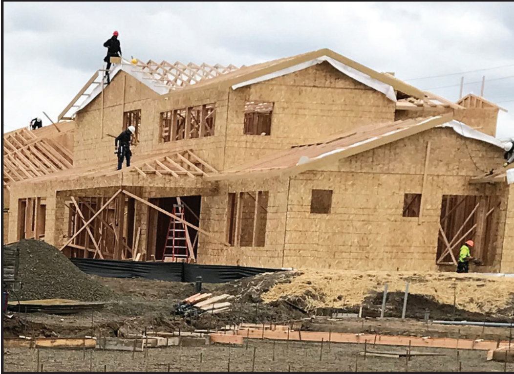
New home construction in the Frog Pond neighborhood.
