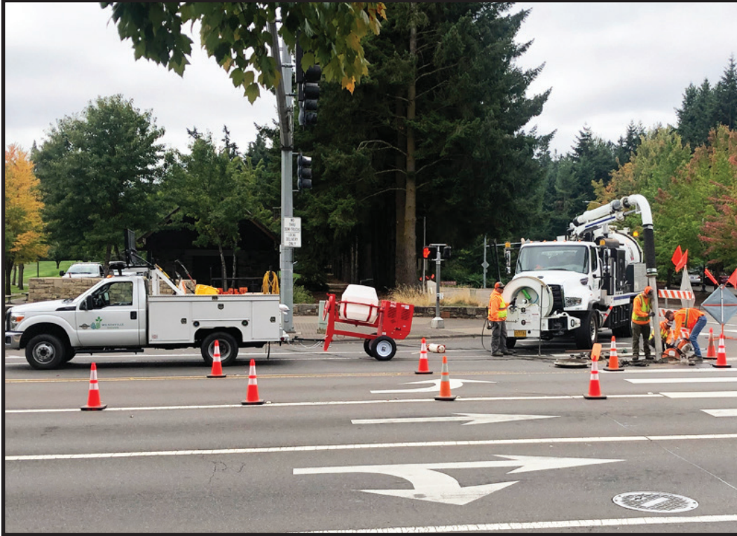
Roads/stormwater crew repairing a manhole on Wilsonville Road.
