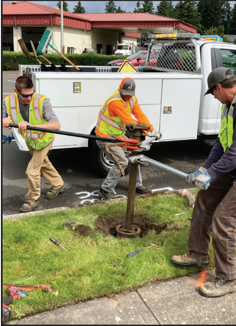
Water crew exercising a valve.
