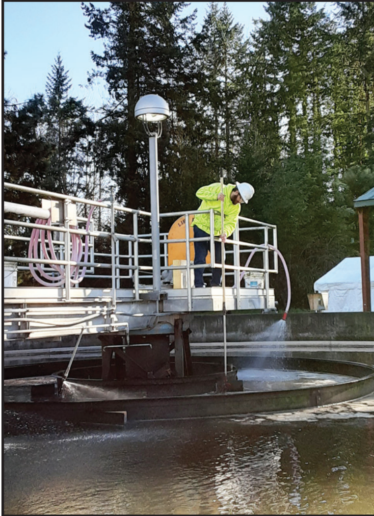
Jacobs Company staff cleaning clarifier.
