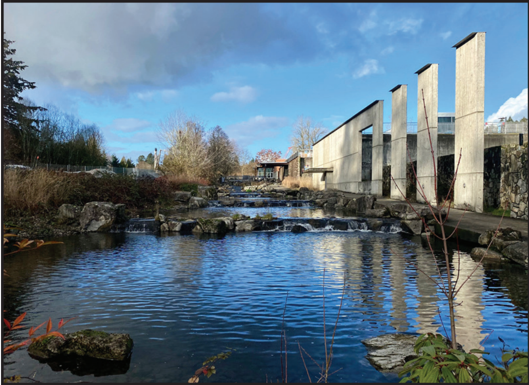
Wilsonville Water Treatment Plant. Photo Credit: Susan Reep.
