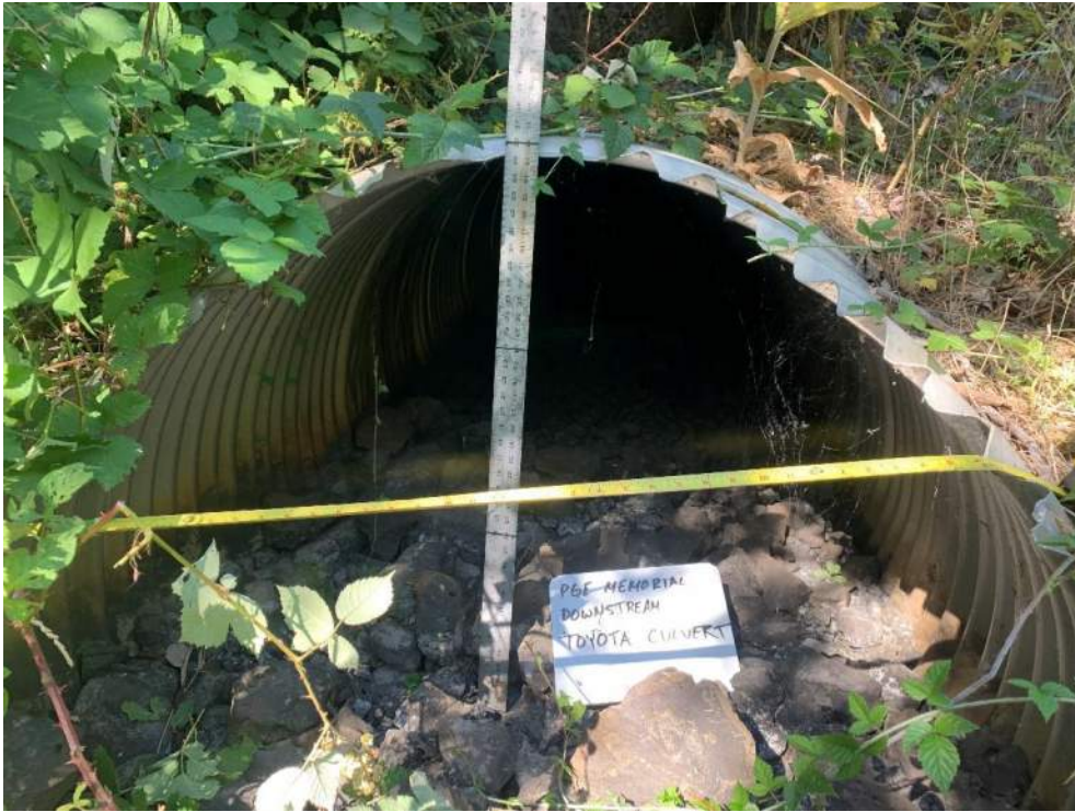
Photo 11: East side of 54-inch culvert surrounded with rip rap and invasive species.
