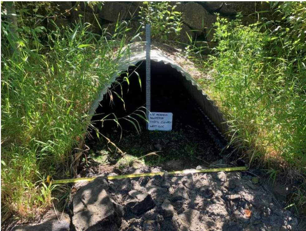
Photo 12.A: West side of 54-inch culvert.
