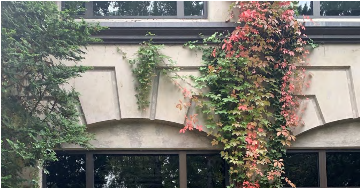
An office development with stained walls by the owners in Bellevue, WA from 1998 (permitted as I-90 1997). I include this close-up view from 2021 to show the nicely patinaed stained pre-cast concrete after weathering for 34 years. The vines have been cut back a few times to control them and the stain holds up very well. This was the first successful stained project by the owners after previous attempts ended being painted. I check every few years to verify if the sealer is still functioning, and irrigation spray still beads up on the walls! Shell architect is LMA. Address: 15405 SE 37th Street, Bellevue, WA 98006
