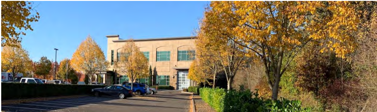
Two views of W3 in Wilsonville from 2012, the last part of the complex that includes W1 and W2 and borders the SROZ. Originally expansion space for DWFRITZ, it is now occupied by Sig Sauer, Electro-Optics. This wall stain is another warm example, and the warm afternoon sunlight is an influence. Shell architect is LMA. Address: 27100 SW Parkway Ave, Wilsonville, OR 97070
