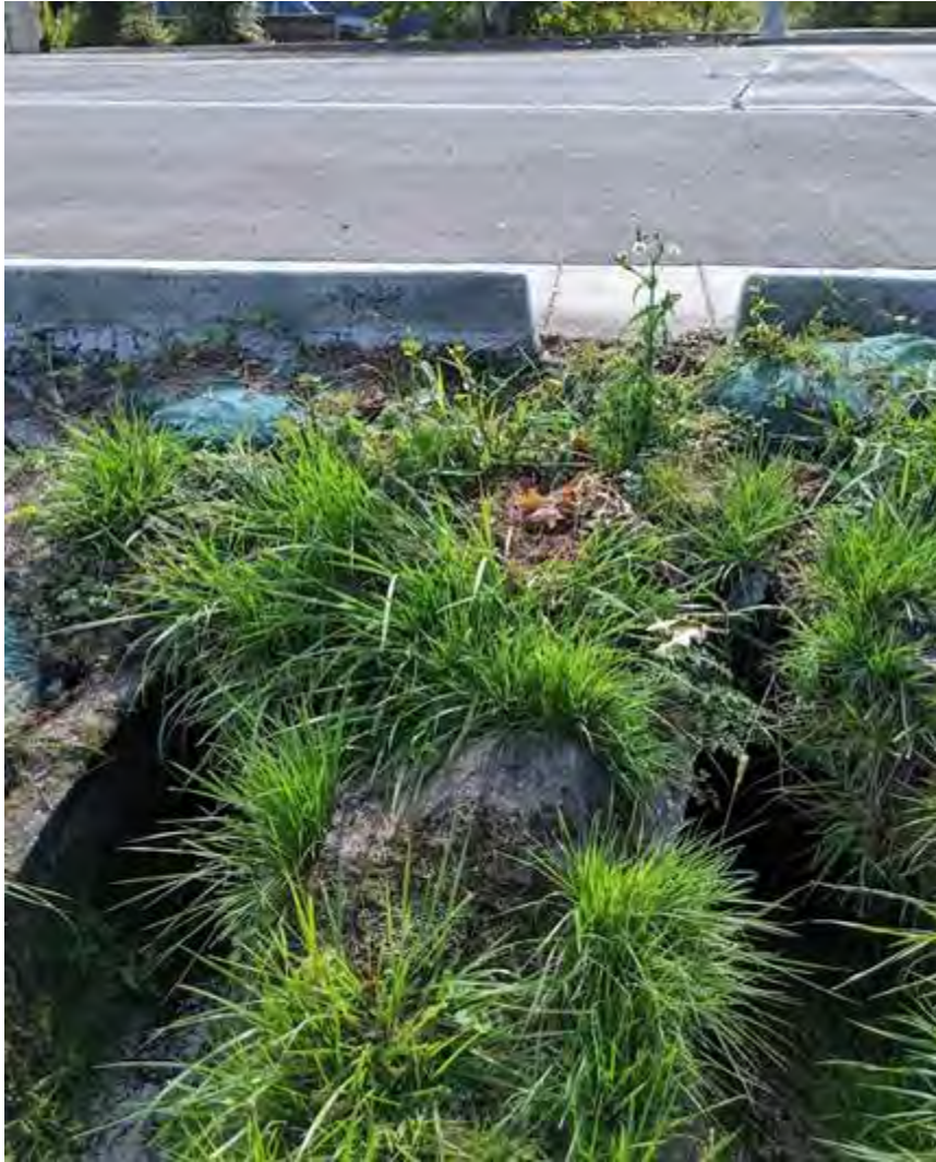
Image 2 – Existing 18" Culverts under SW Boeckman Road
