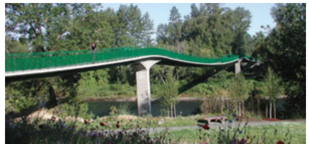
Rogue River Pedestrian Bridge, Grants Pass, OR
