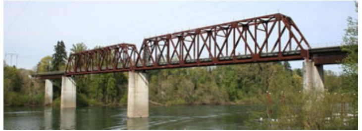
Portland and Western Railroad Bridge, Wilsonville, OR
