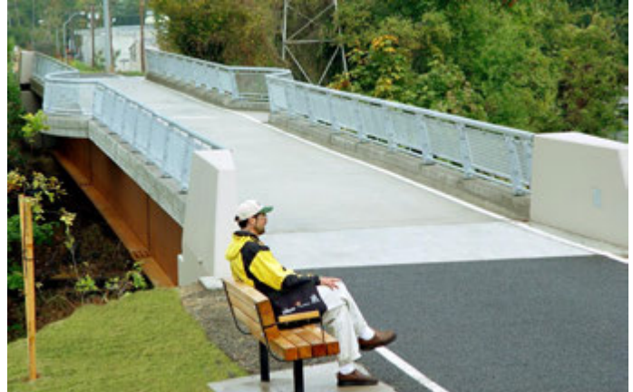
Springwater Trail Bridges: Johnson Creek Crossing, Portland, OR
