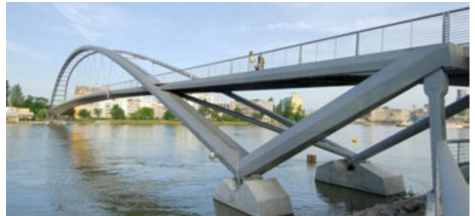
Three Countries Pedestrian Bridge, Germany, Switzerland, France
