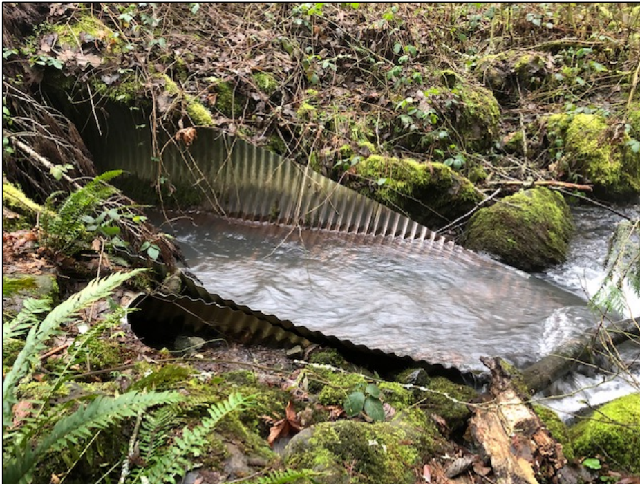
Main Large Corrugated Metal Pipe (CMP) Culvert conveys creek flows under the Road
