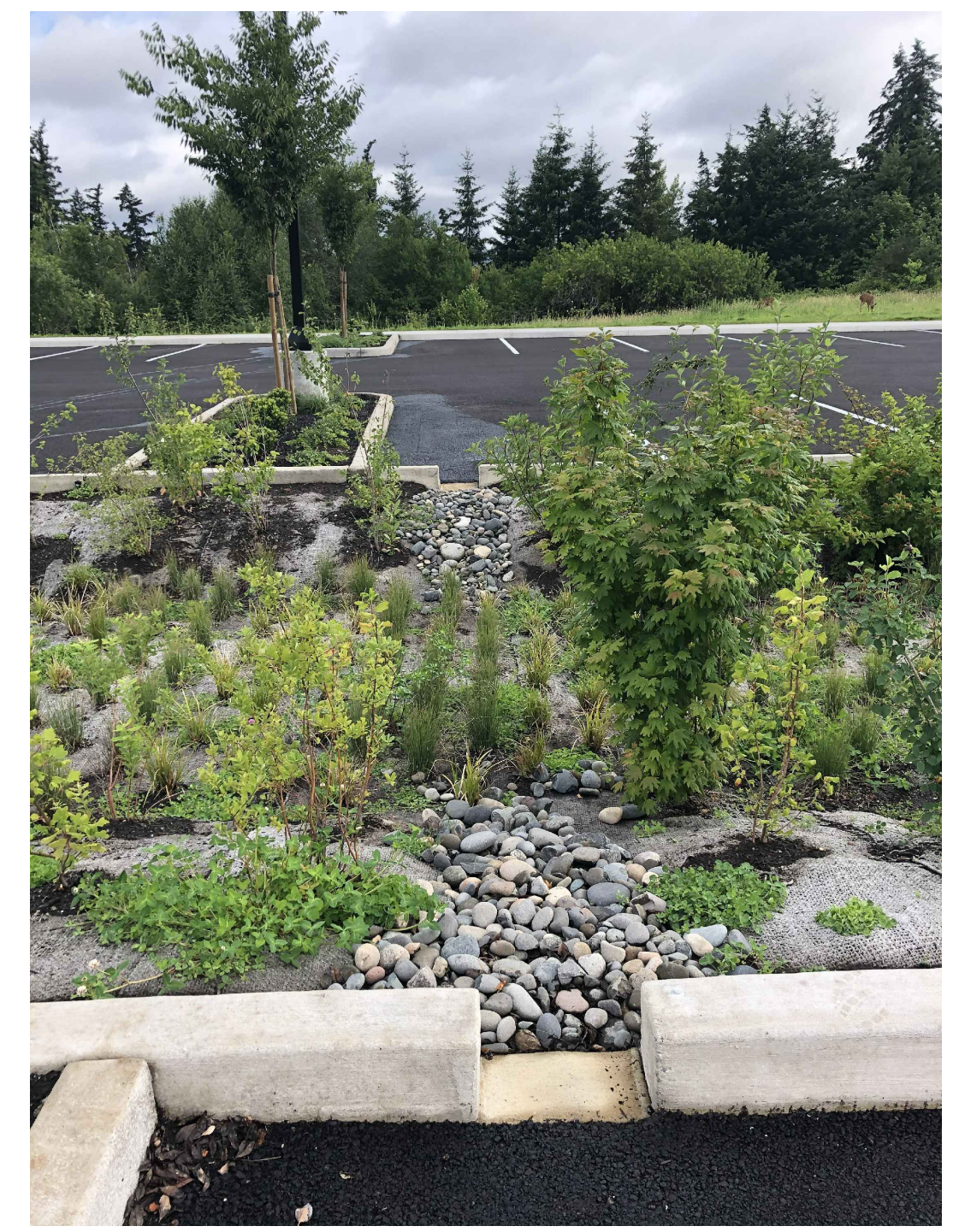
TYPICAL BIOSWALE PLANTING
