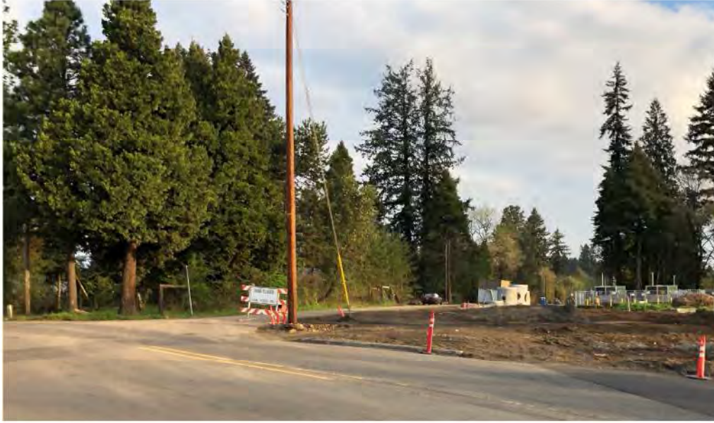
FIGURE 5: CURRENT CONSTRUCTION AT GARDEN ACRES ROAD/CLUTTER STREET/RIDDER ROAD
