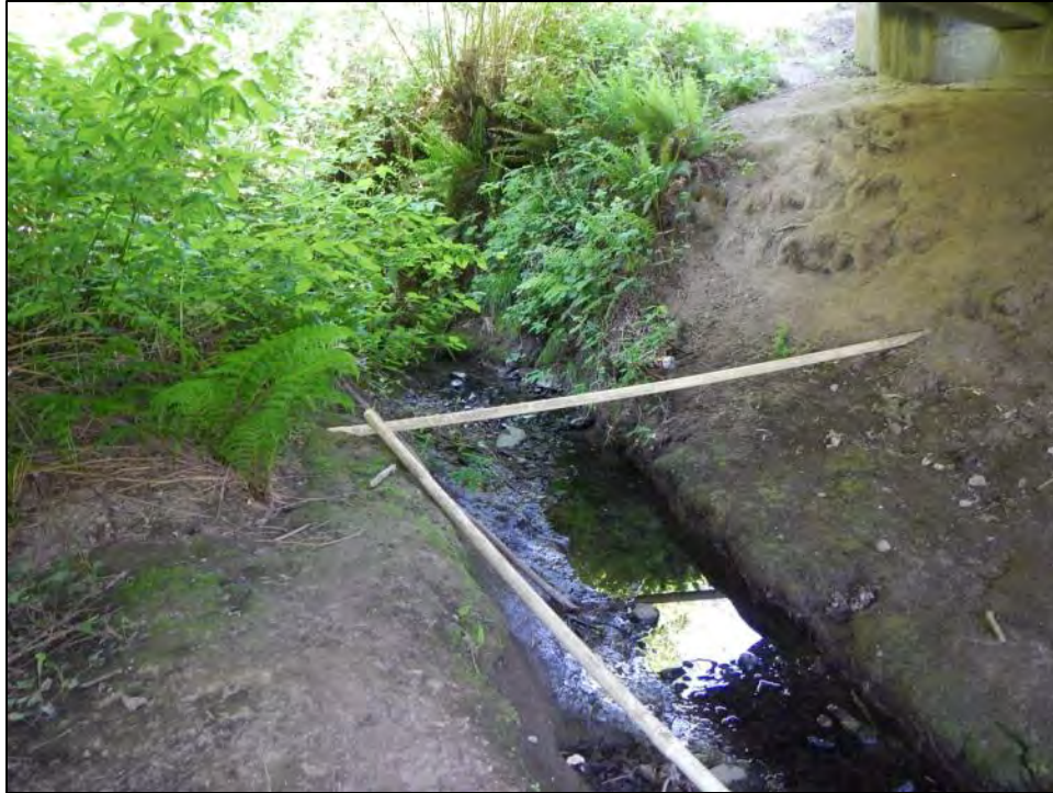
Photo 3: Looking north at Arrowhead Creek from under the bridge (May 8, 2015).
