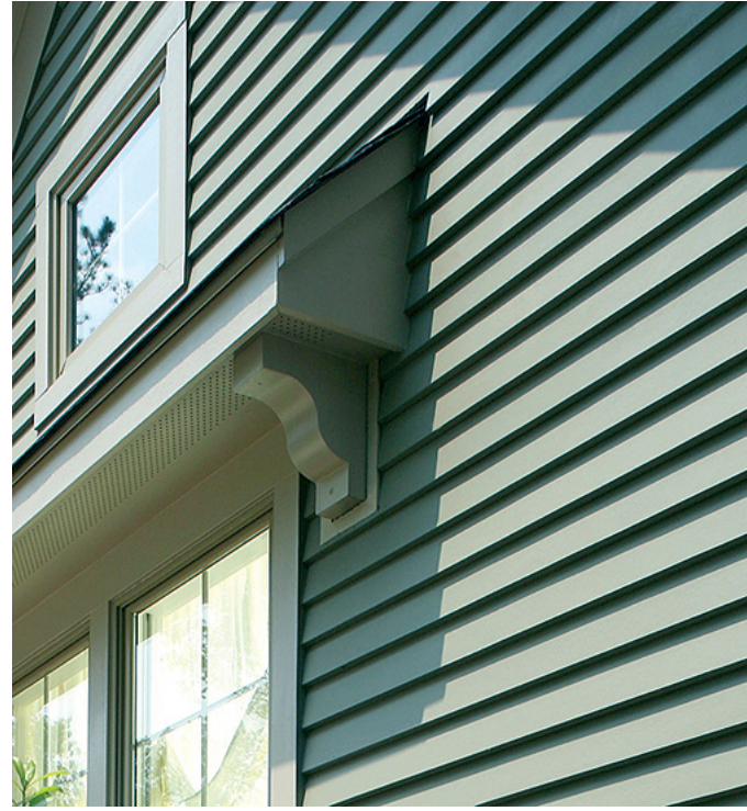
Fiber Cement Lap Siding
