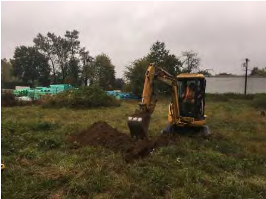
Test Pit TP-3
