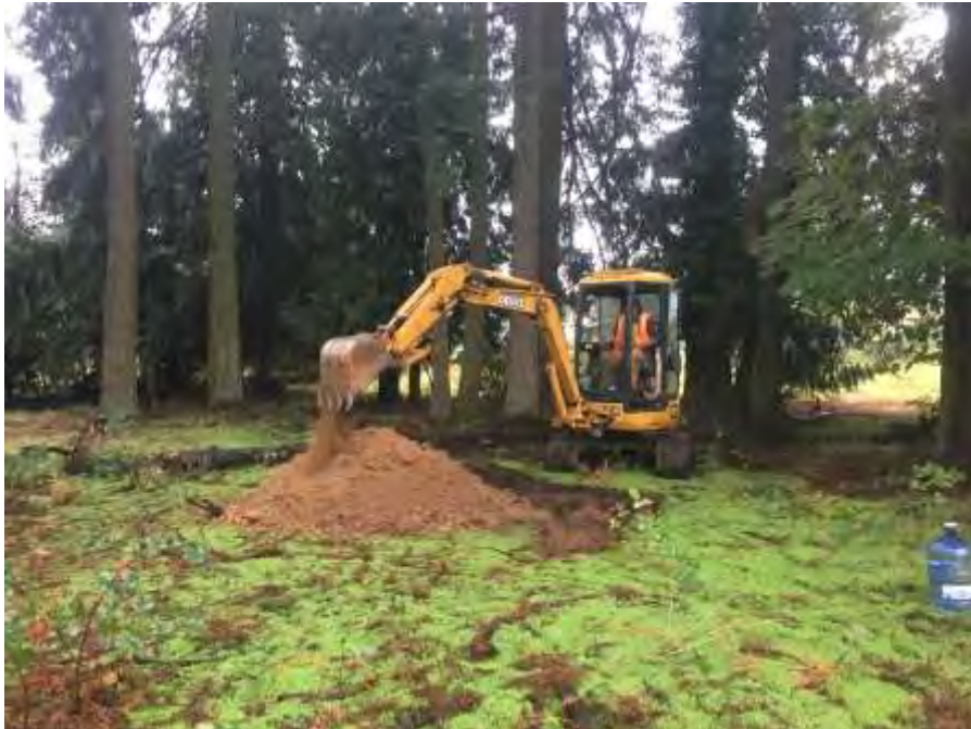
Test Pit TP-1
