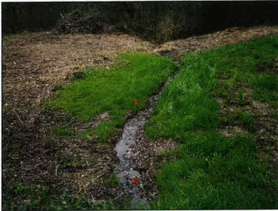
Photo O. View west of Swale C as it becomes Tributary 1 in the ravine. Photo date April 5, 2017.
