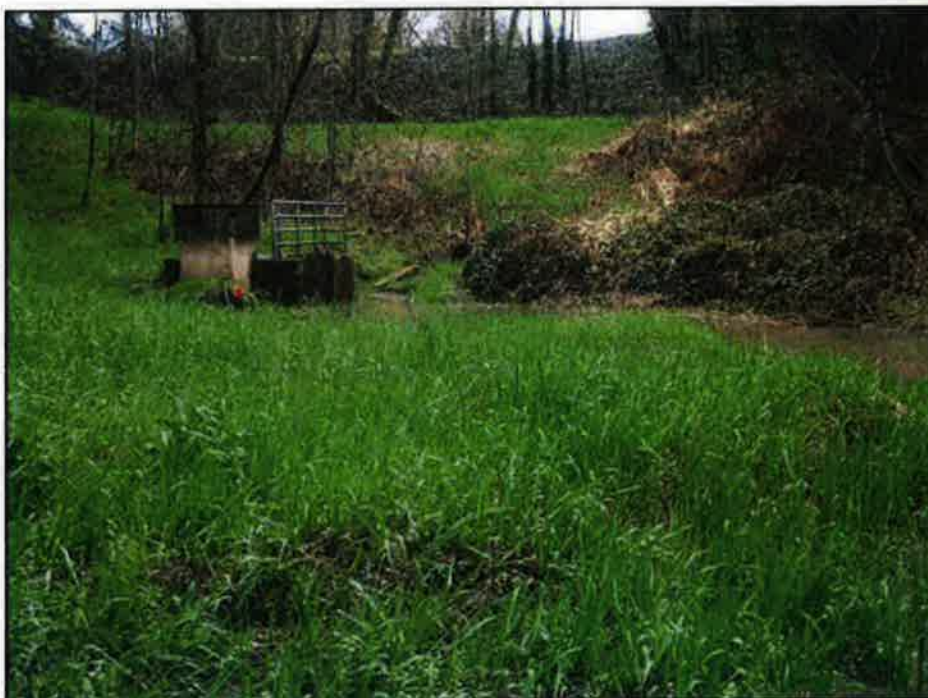
Photo D. View south of concrete drain structure. Photo date March 24, 2017.
