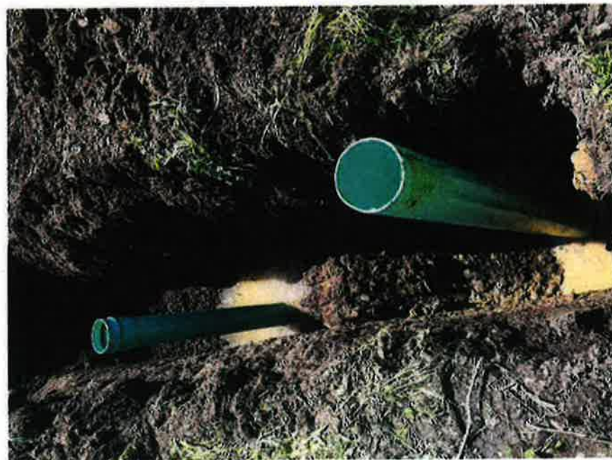
Infiltration Testing in Test Pit TP-1
