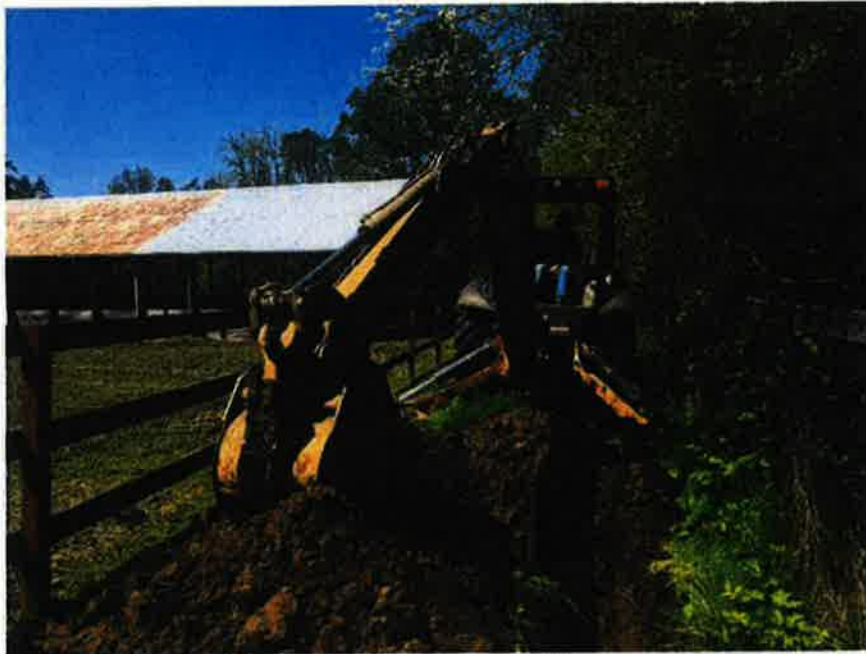
Excavation of Test Pit TP-5 (View to North)
