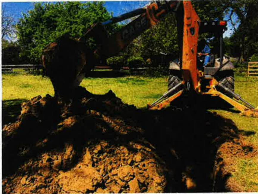
Excavation of Test Pit TP-7 (View to North)
