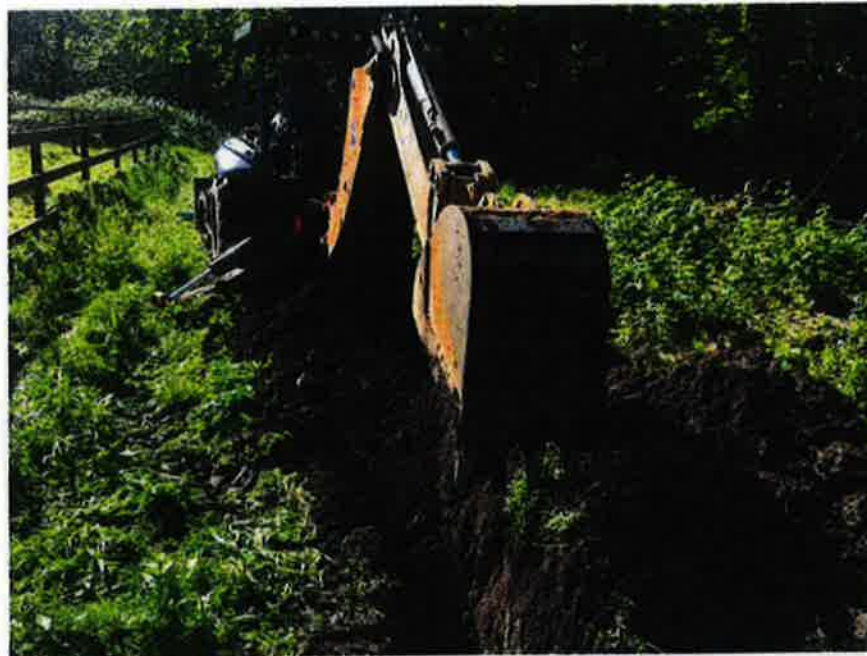
Excavation of Test Pit TP-1 (View to Southeast)
