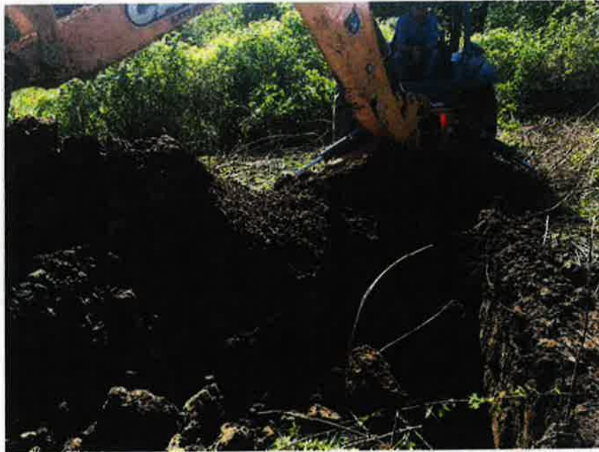
Excavation of Test Pit TP-10 (View to North)
