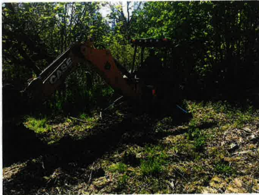
Excavation of Test Pit TP-8 (View to West)
