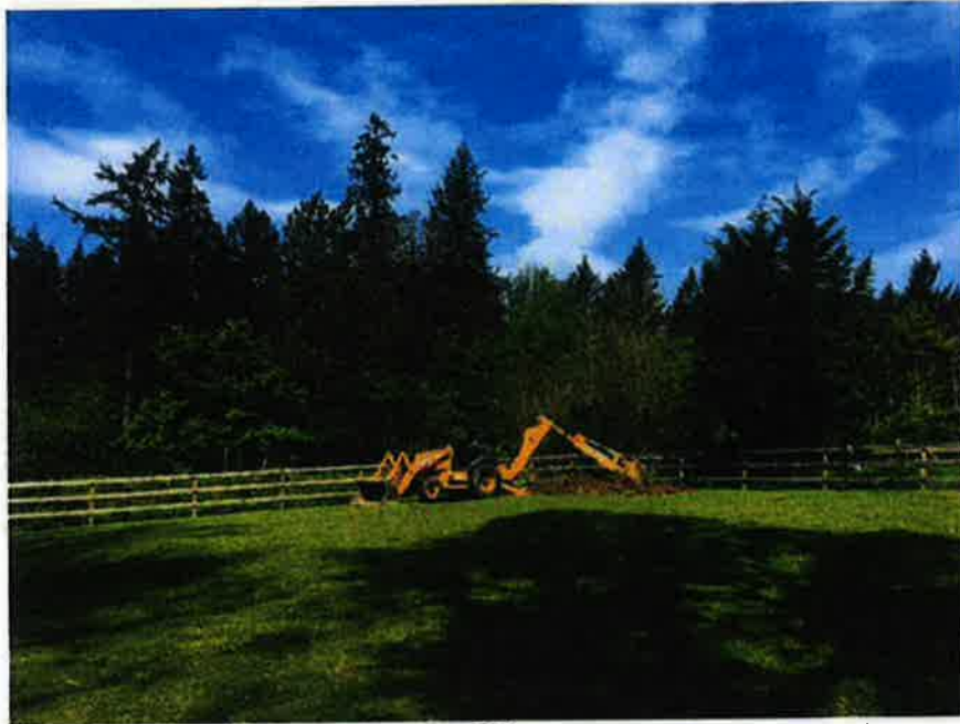
Excavation of Test Pit TP-2 (View to Northwest)
