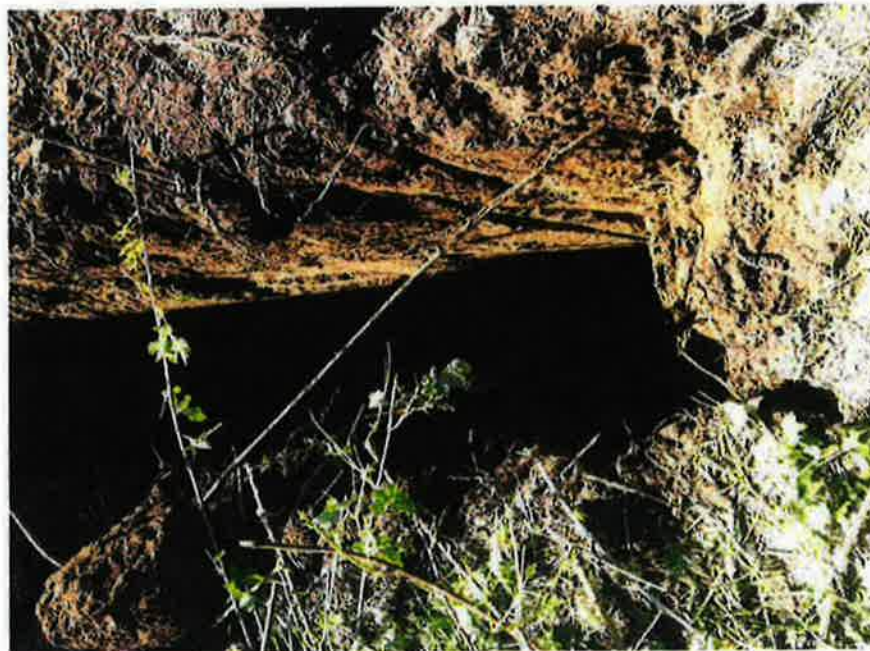
Test Pit TP-10
