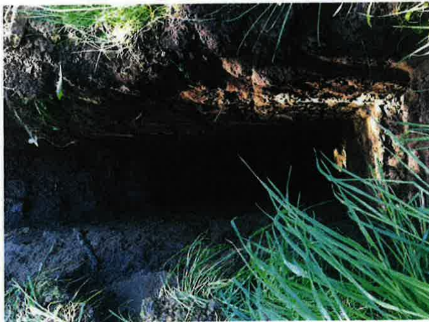
Test Pit TP-9
