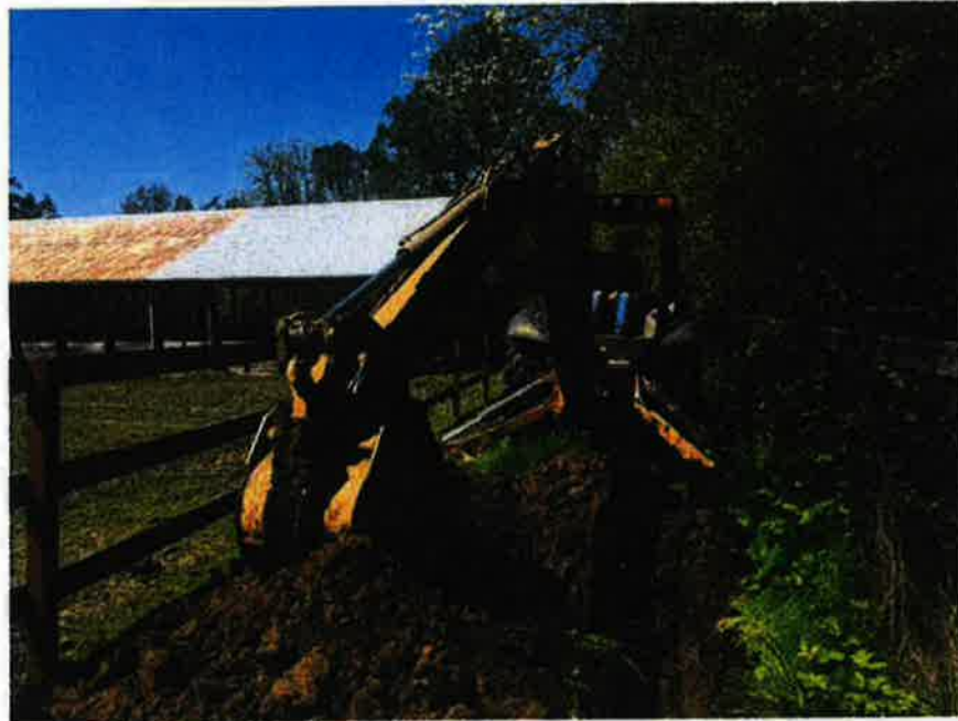
Excavation of Test Pit TP-4 (View to West)
