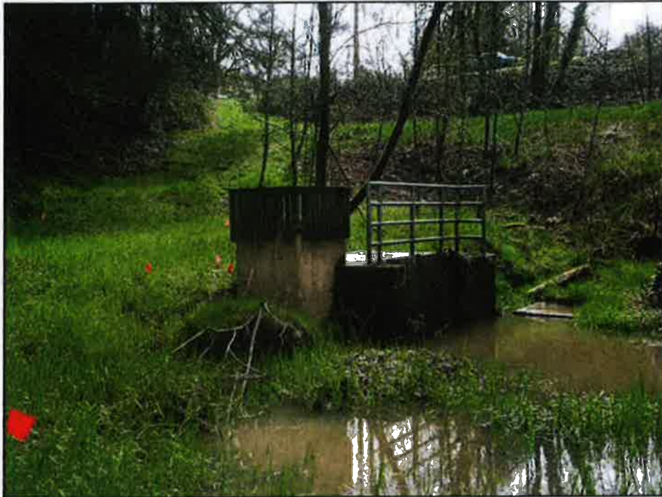
Photo E. Close up of concrete drain structure. Photo date March 24, 2017.
