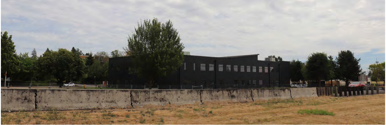
Figure 13 - I-5 South Current Condition
