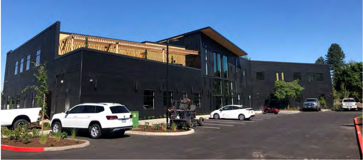
Finished building – July 2020
