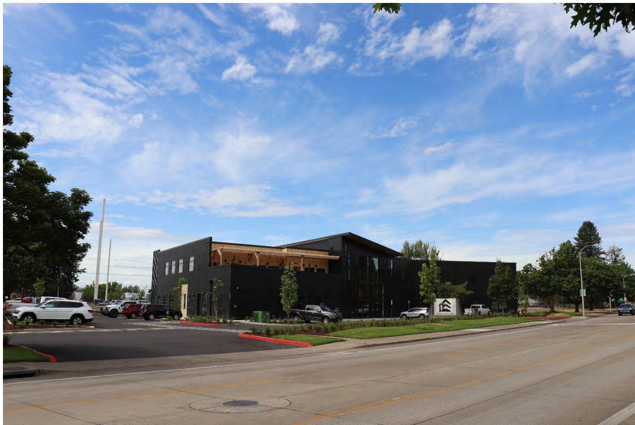
Figure 1 – Current Condition of Building
