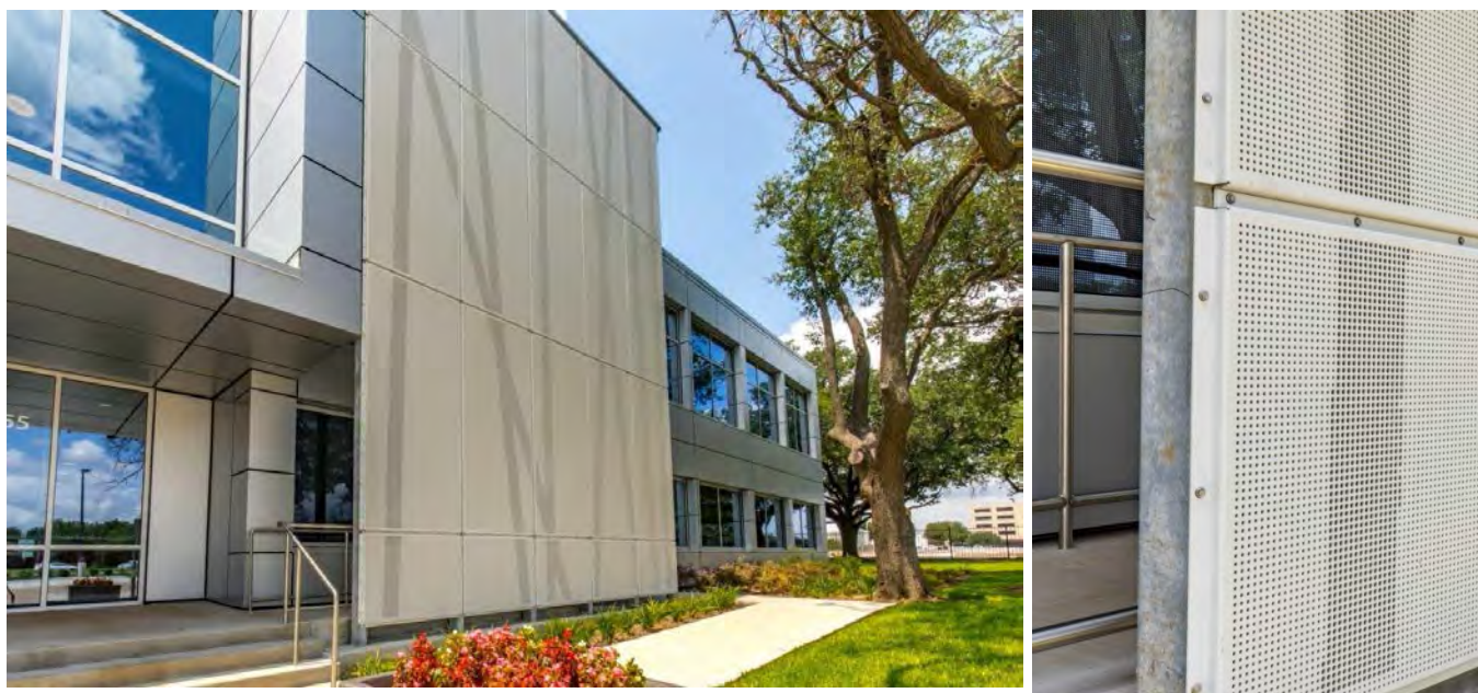
Figure 7 - Hendrick Corp Project in Dallas, TX
