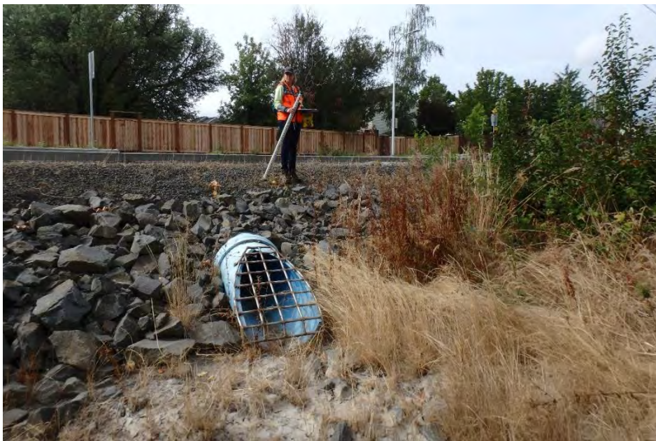
Figure 14. Upstream end of culvert under SW Advance Road
