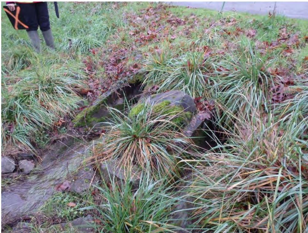
Photo 2 Upstream Ends of Culverts
