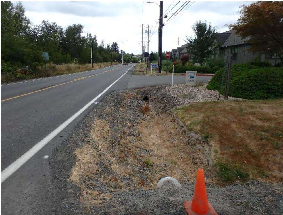
Figure 10. West ditch at church property with gravel and less vegetation, 2 ft depth, 2 ft bottom width and 2:1 side slopes, upstream of driveway crossing (Node 27).
