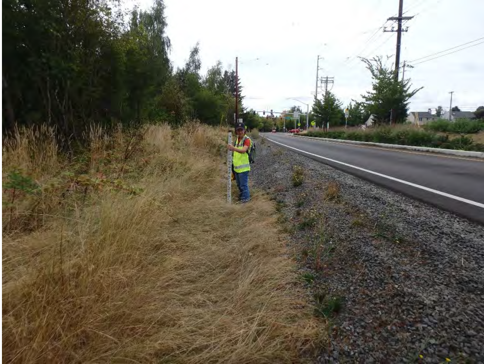
Figure 7. East ditch with 3 ft bottom width downstream of elevation change (downstream of Node 9)
