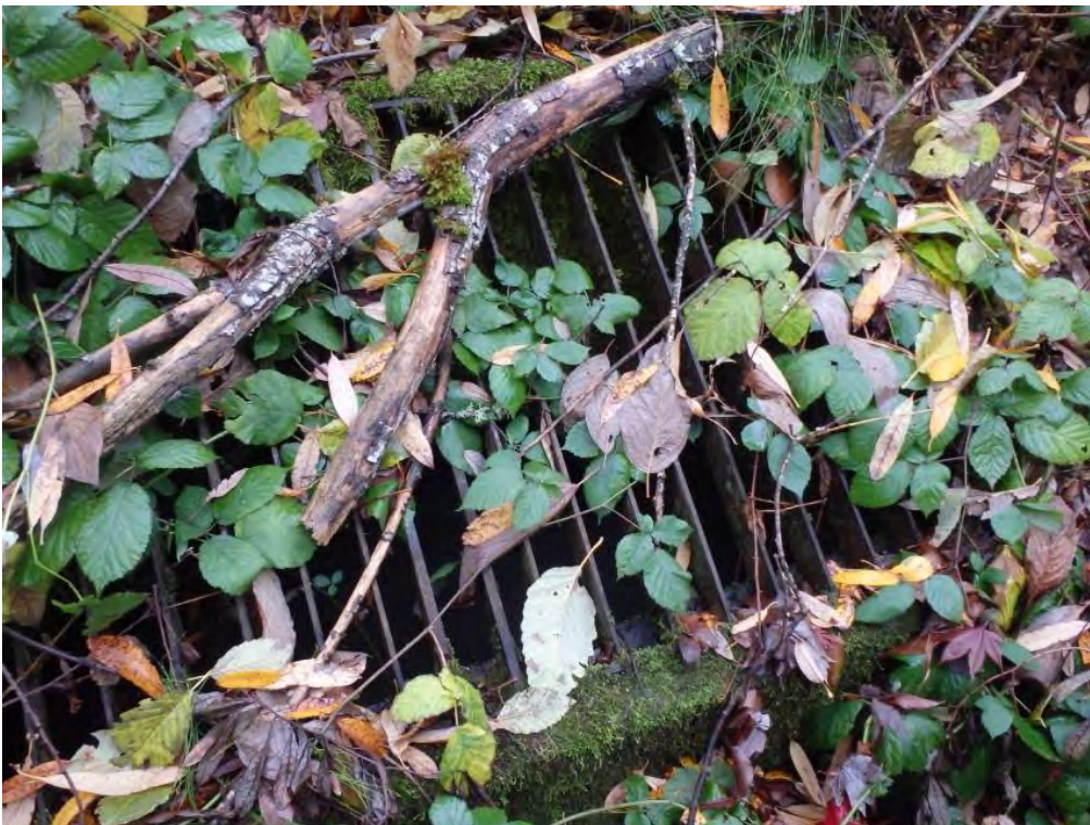
Photo 8 36-inch Outfall into Concrete Box
