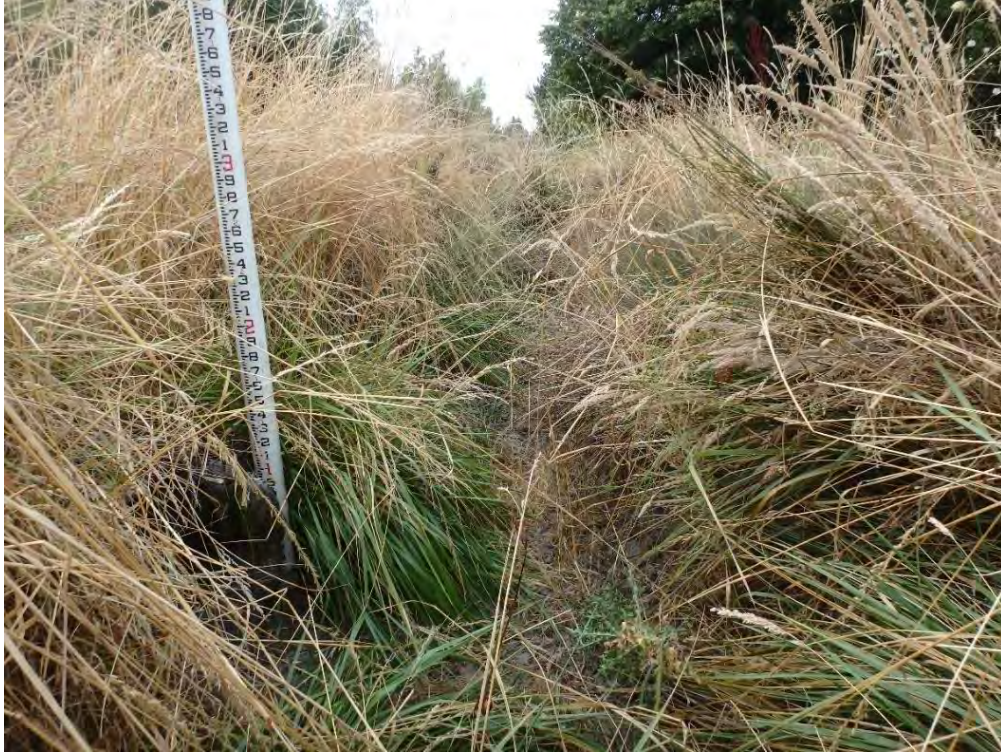
Figure 1. Upstream end of 15" culvert in west ditch (Node 2)
