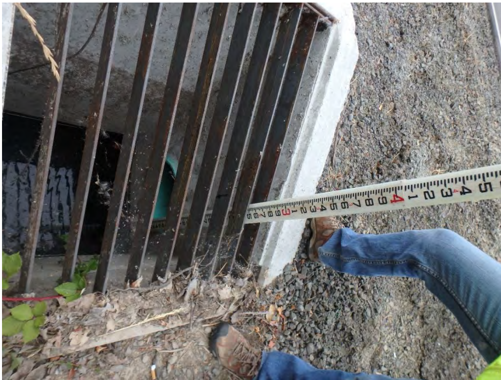
Figure 8. East ditch inlet with pipe out to the west (node 10)
