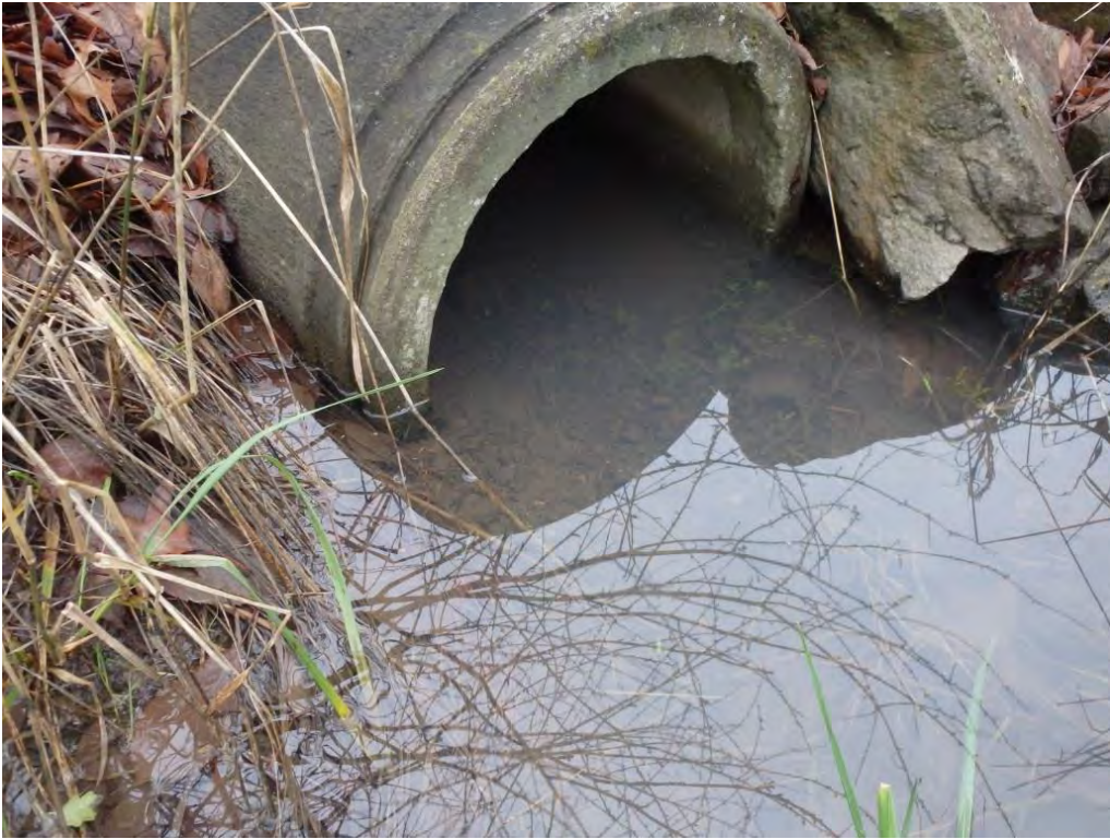
Photo 3 Downstream of culvert with gravel accumulation
