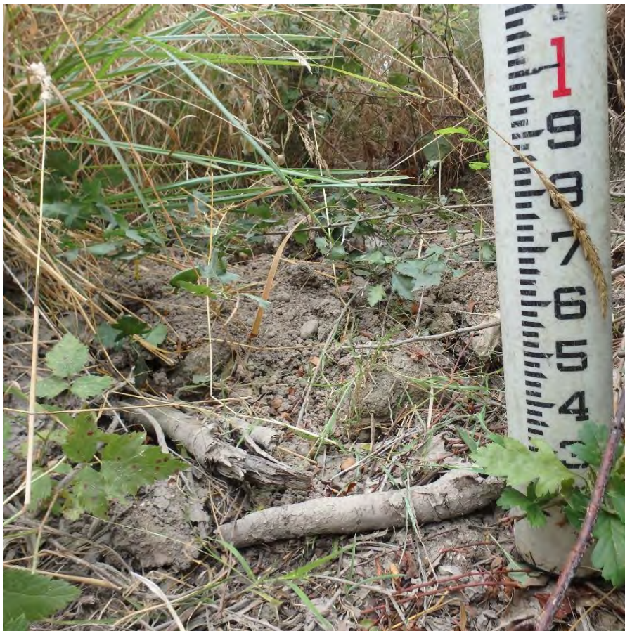
Figure 6. Debris and sedimentation raises channel bottom 0.8 ft. (Node 9)
