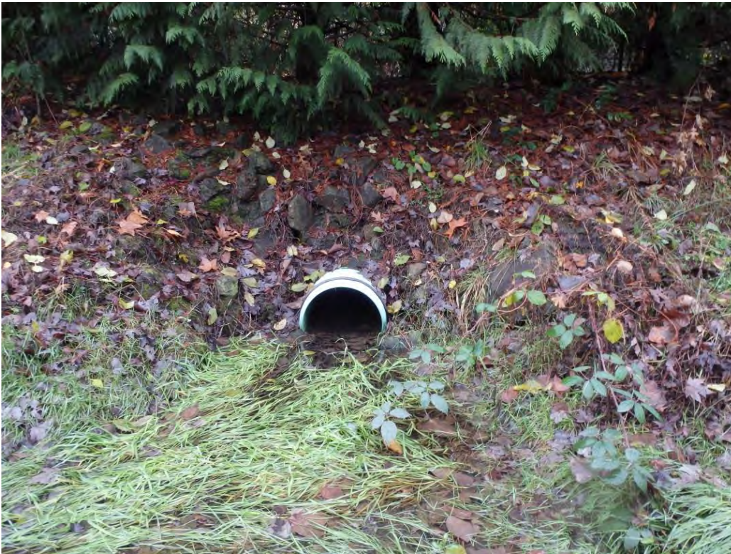
Photo 6 Partly submerged 18-inch CCP contributing culvert
