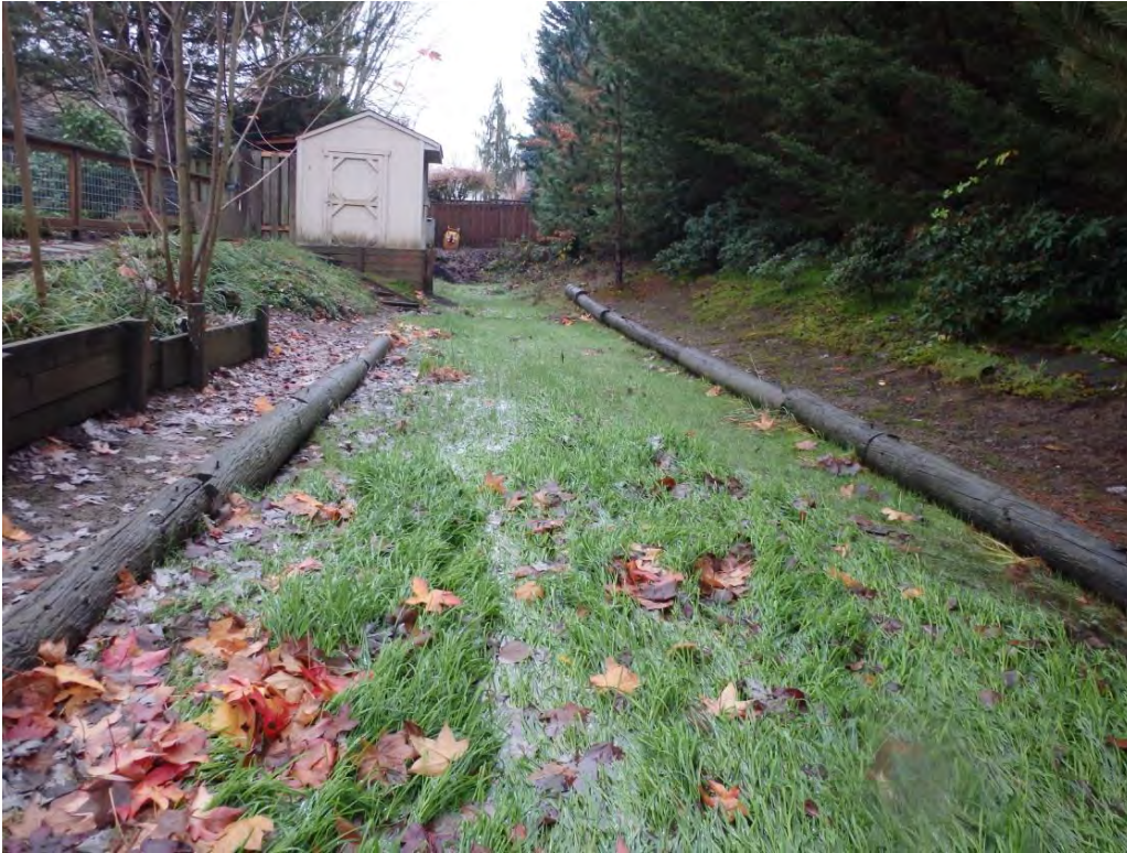
Photo 5 Vegetated channel with taller banks and logs channeling flow
