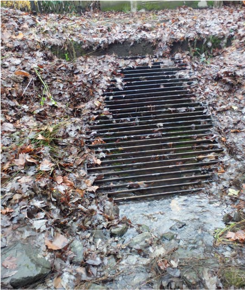
Photo 7 36-inch culvert under SW Willow Creek Drive
