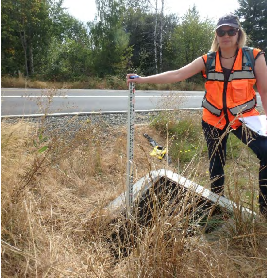
Figure 13. West ditch collected in inlet directly downstream of outfall from church swale. Pipe out to east and connects with discharge from east ditch in manhole and continues south.
