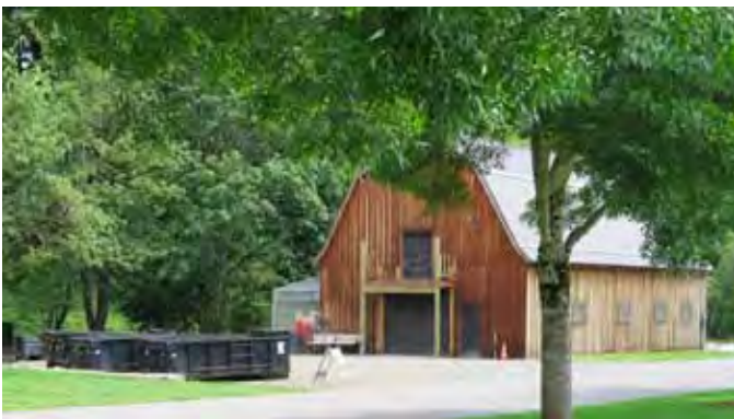
Future Picnic Shelter with Restroom
