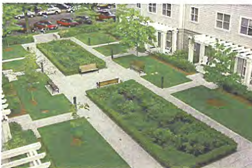
Stormwater Planter / Infiltration Garden Portland, Oregon
