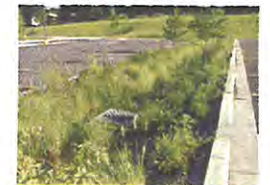
Bio-retention Cell with Amended Soils Prince George's Sound, Maryland Photo: PGS
