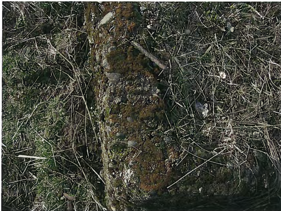
Close up of concrete matrix of the foundation.
