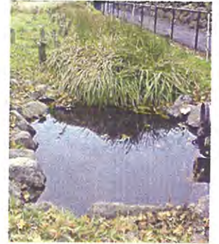
Vegetative Swale w/ Forebay Washington Co., Oregon Photo: AEI
