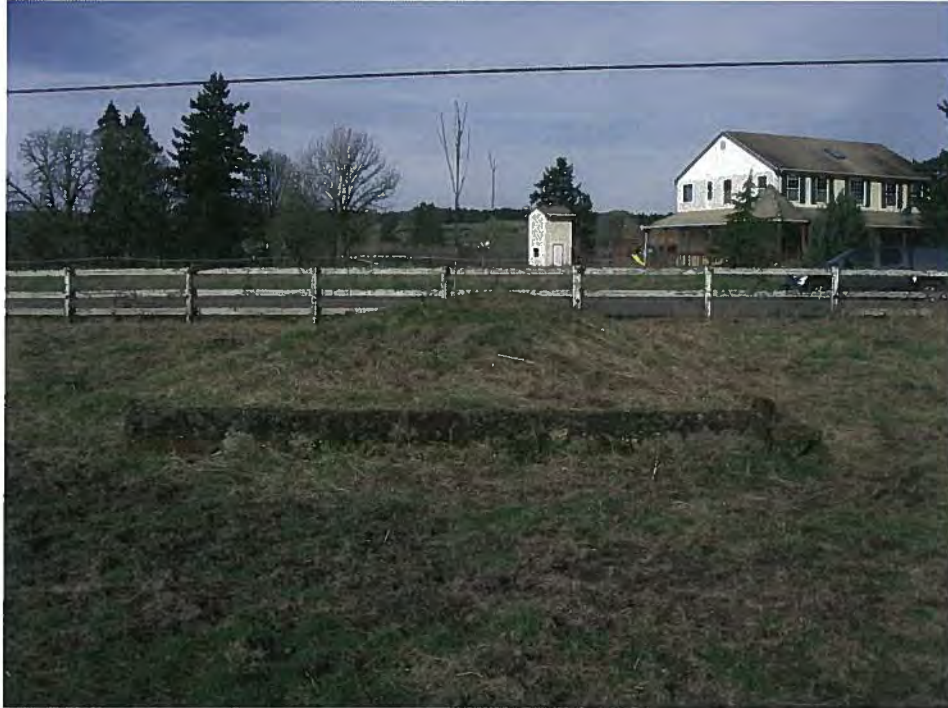
Overview of foundation, view to the west.
