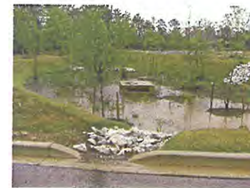
Bio-retention Cell with Amended Soils Prince George's Sound, Maryland
