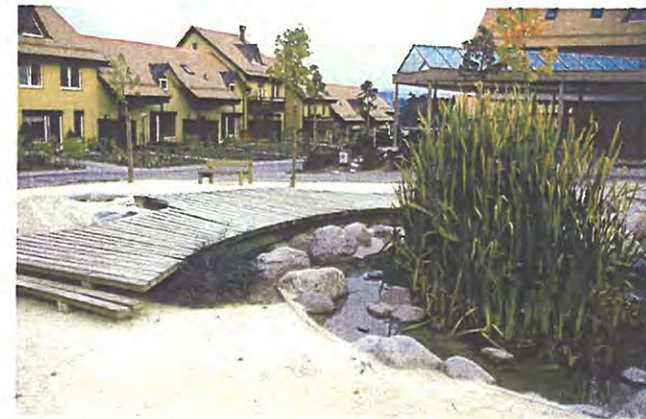
Rainwater Bioretention Cell. Germany
