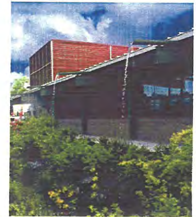
Vegetative Filter at BES Water Quality Lab, City of Portland
