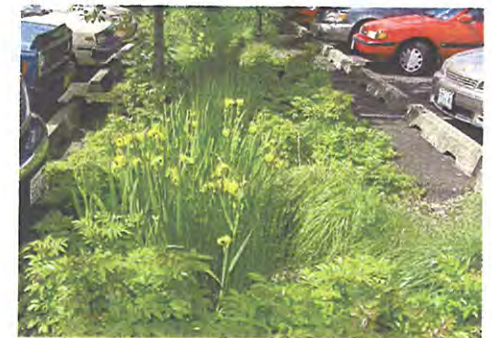
Vegetative Swale Portland, Oregon
