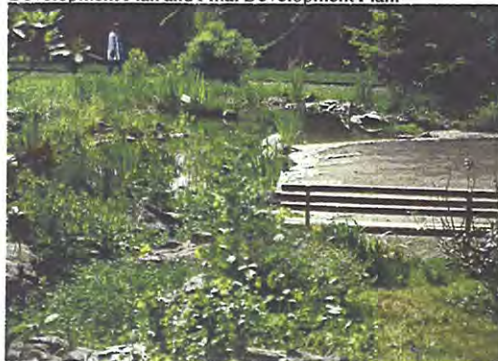
Detention Pool and Bio-swale in Park, Germany Photo: DA
