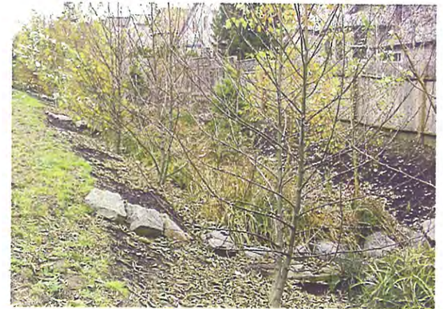
Vegetative Swale with Check Dams Washington Co., Oregon Photo: AEI
