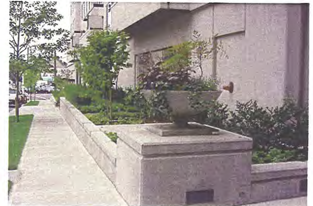
Stormwater Planter Portland, Oregon
