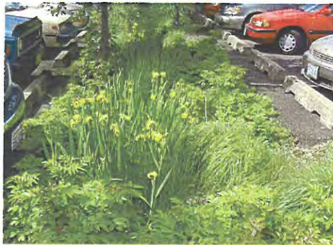
Bioretention Cell, OMSI, City of Portland
