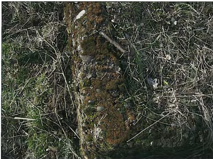
Figure 13. Close-up of concrete matrix of the foundation.
