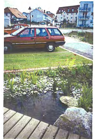
Permeable Pavers and Bioretention Cell Photo: DA Germany
