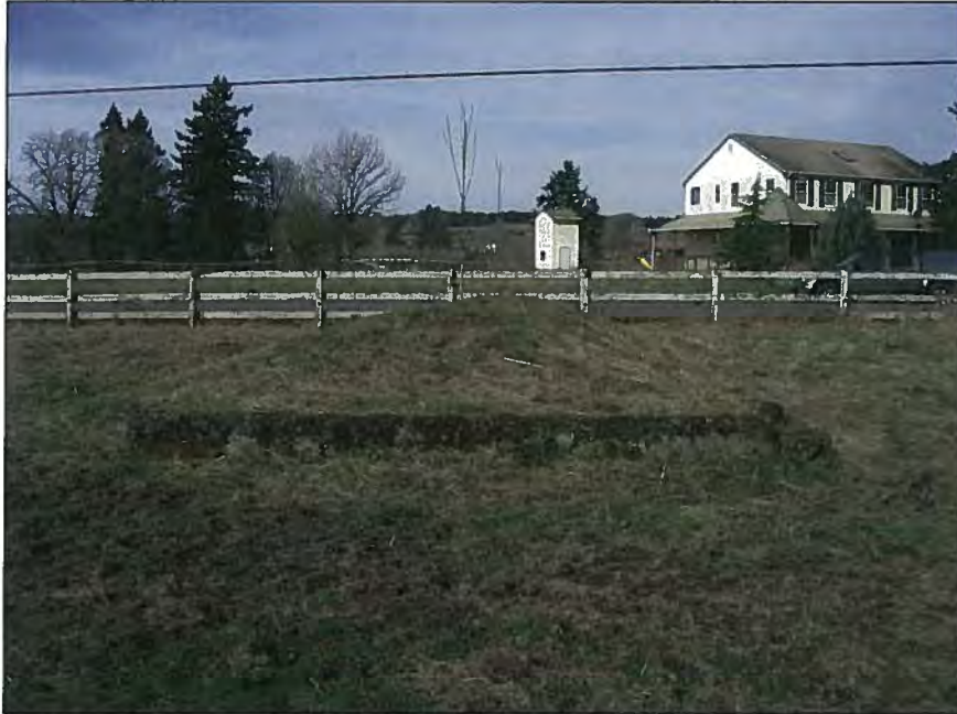
Figure 12. Overview of foundation, view to the west.
