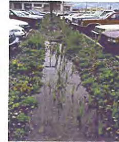
Rainwater Bioretention Cell, OMSI, Portland, Oregon Photo: BES
