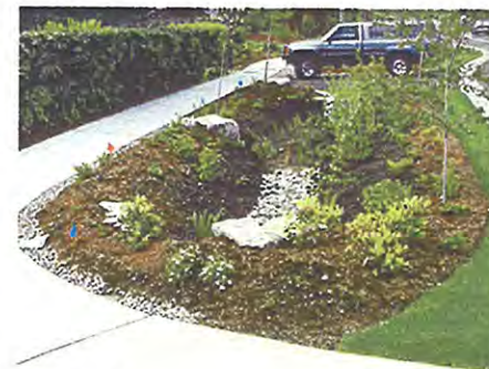
Bioretention Cell Seattle, Washington
