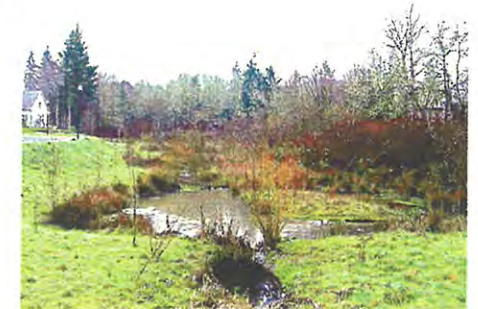
Bioretention Pond, Washington Co. Oregon
