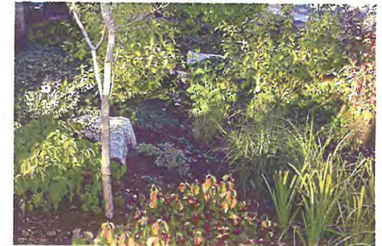
Rainwater Bio-retention Cell, with Amended Soils Street Edge Alternative, Seattle, Washington
