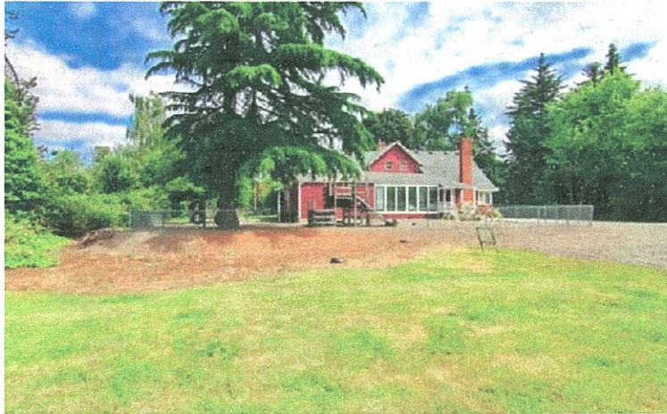
Figure 4. Back View of the Property including parking area and new location of access / driveway
