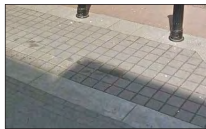
PERMEABLE CONCRETE UNIT PAVERS AT ON-STREET PARKING STALLS MANUFACTURER: WILLAMETTE GRAYSTONE MODEL: AQUAPAVE PERMEABLE CONCRETE PAVER COLOR: GRAY FINISH: STACKED SIZE: 9.5 X 9.5" X 80MM
