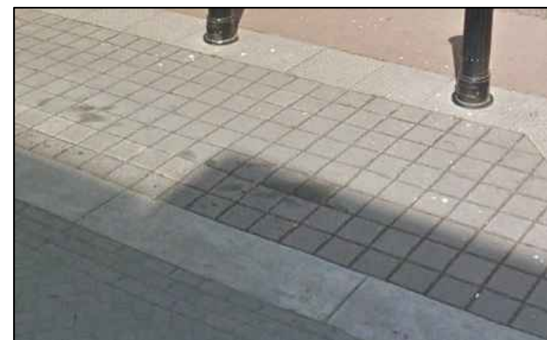
PERMEABLE CONCRETE UNIT PAVERS AT ON-STREET PARKING STALLS MANUFACTURER: WILLAMETTE GRAYSTONE MODEL: AQUAPAVE PERMEABLE CONCRETE PAVER COLOR: GRAY FINISH: STACKED SIZE: 9.5 X 9.5" X 80MM
