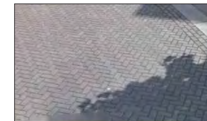
PERMEABLE CONCRETE UNIT PAVERS AT VEHICULAR AREAS MANUFACTURER: WILLAMETTE GRAYSTONE MODEL: AQUAPAVE PERMEABLE CONCRETE PAVER COLOR: CHARCOAL FINISH: CENTURY SIZE: 5" X 10" X 80MM - HARRINGBONE PATTERN
