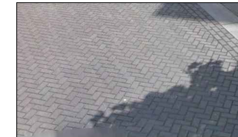
PERMEABLE CONCRETE UNIT PAVERS AT VEHICULAR AREAS MANUFACTURER: WILLAMETTE GRAYSTONE MODEL: AQUAPAVE PERMEABLE CONCRETE PAVER COLOR: CHARCOAL FINISH: CENTURY SIZE: 5" X 10" X 80MM - HARRINGBONE PATTERN
