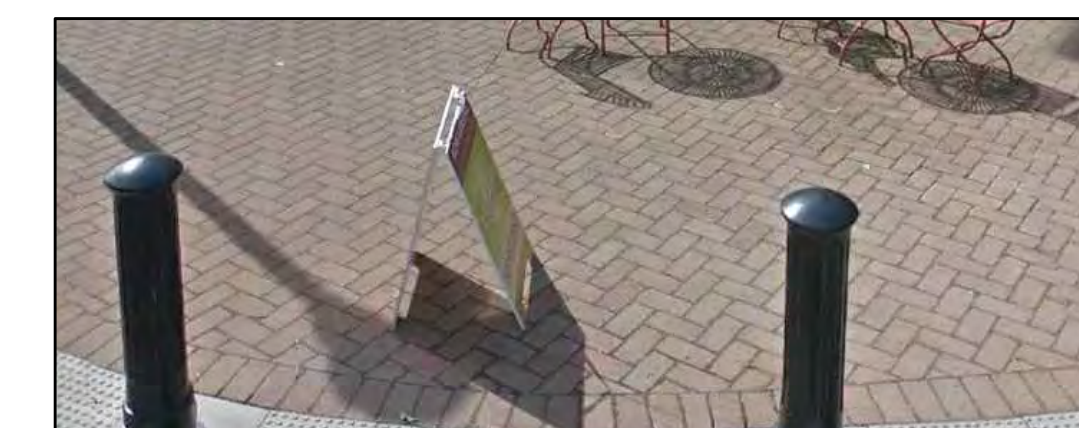
CONCRETE UNIT PAVERS WITH HELL-PROOF POLYMERIC SAND JOINTS MANUFACTURER: WILLAMETTE GRAYSTONE MODEL: AQUABRIC PERMEABLE CONCRETE COLOR: AUTUMN BLEND FINISH: CENTURY SIZE: 5" X 10" X 60MM - HARRINGBONE PATTERN
