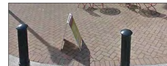
CONCRETE UNIT PAVERS WITH HELL-PROOF POLYMERIC SAND JOINTS MANUFACTURER: WILLAMETTE GRAYSTONE MODEL: AQUABRIC PERMEABLE CONCRETE COLOR: AUTUMN BLEND FINISH: CENTURY SIZE: 5" X 10" X 60MM - HARRINGBONE PATTERN
