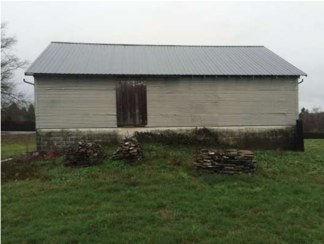
Figure 18: Back (north) elevation.
