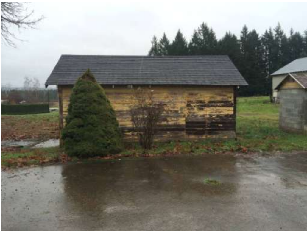
Figure 25: Garage, east elevation.
