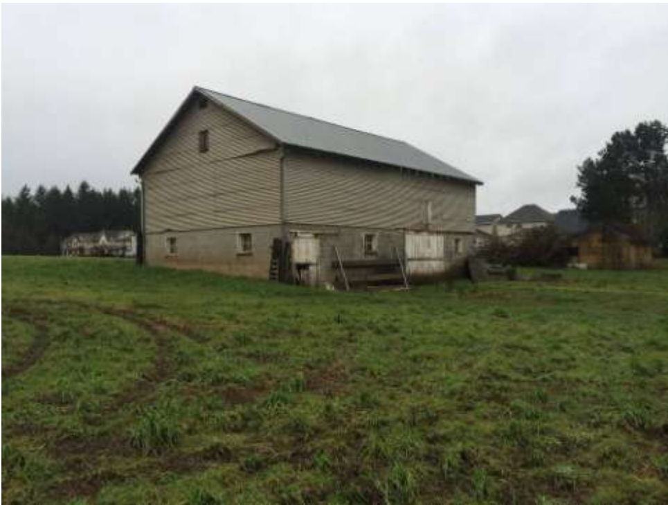
Figure 19: Perspective view, looking at south and west elevations.
