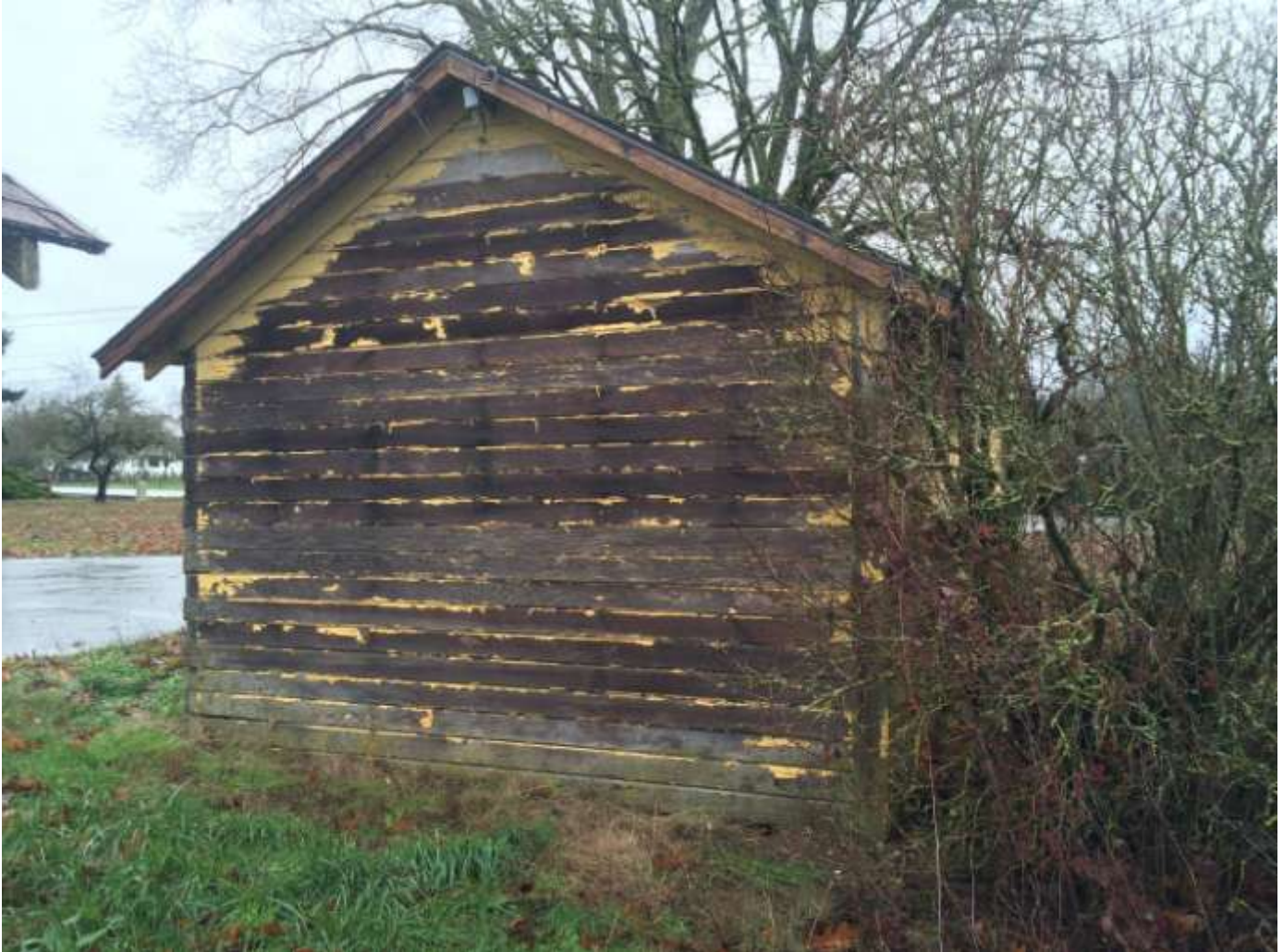
Figure 26: Back, north elevation.
