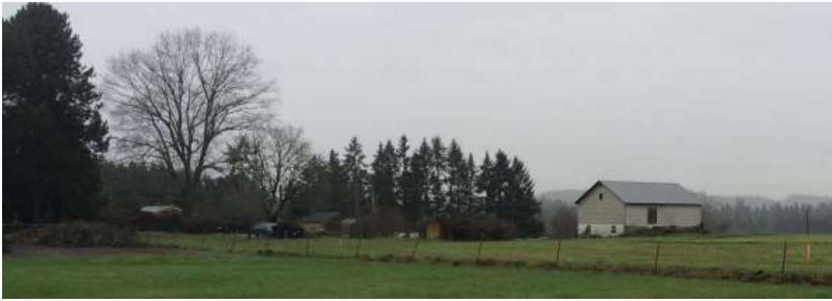
Figure 7: View of Bishoff buildings from the southeast.
