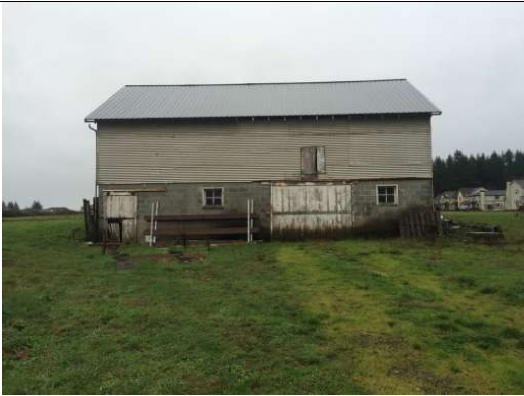
Figure 16: Barn, facade (south) elevation.
