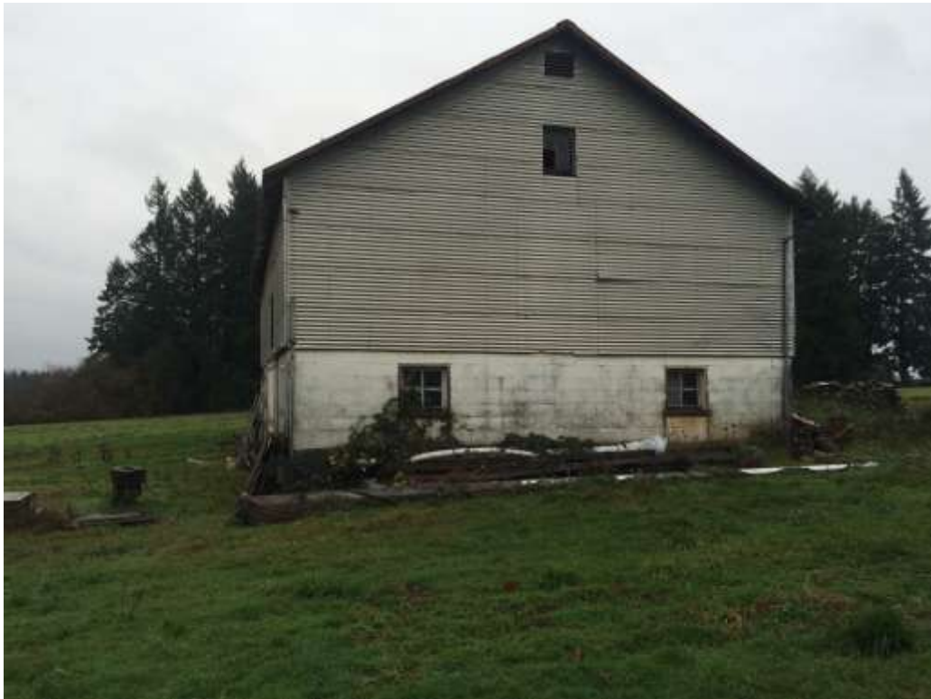
Figure 17: Barn, east elevation.
