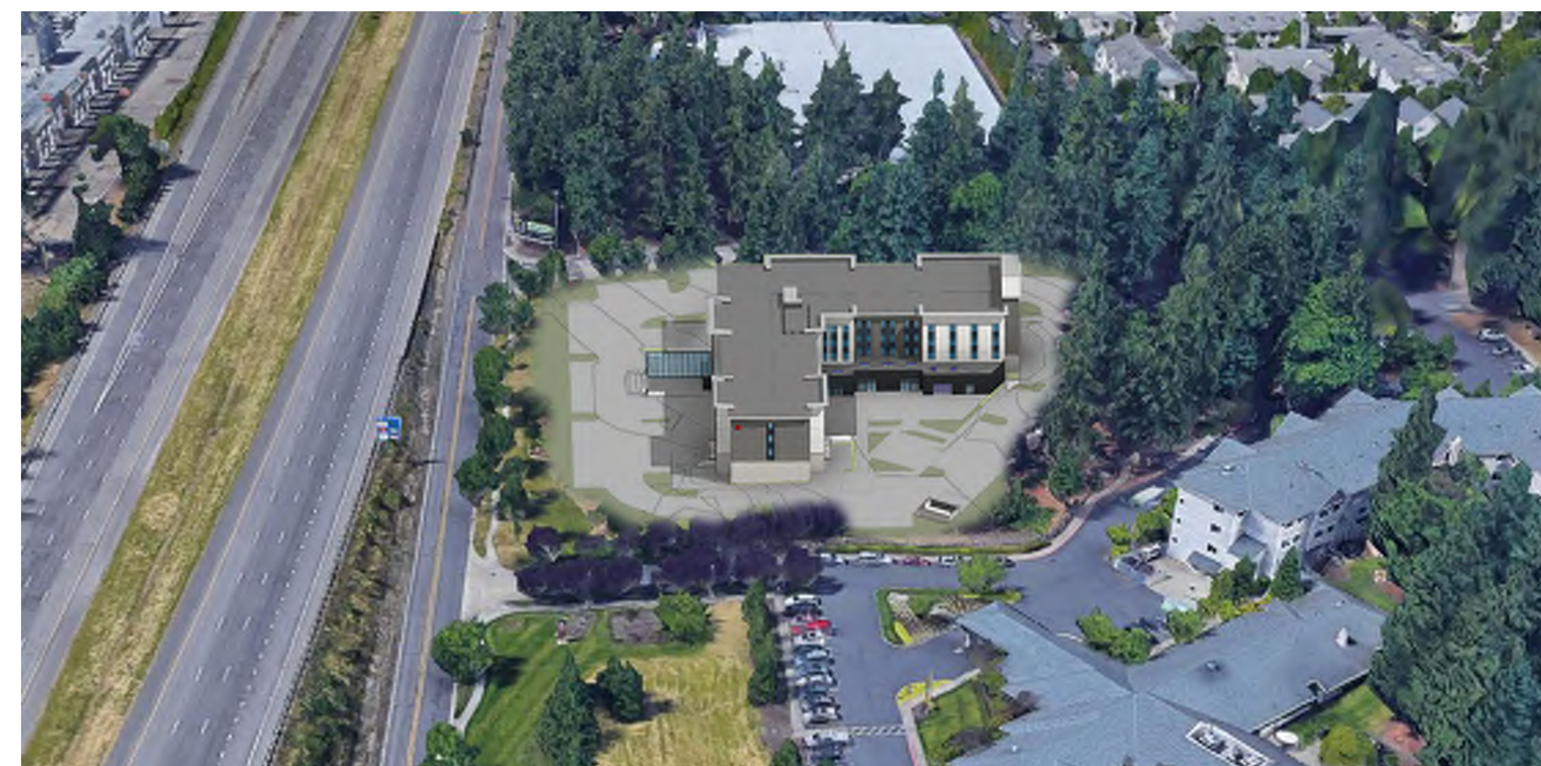
4 BUILDING IMAGE - AERIAL SCALE: 12" = 1'-0"
