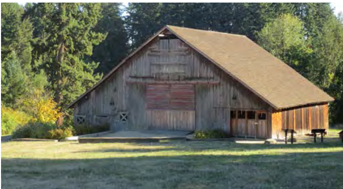
Stein-Boozier Barn - Access Improvements
