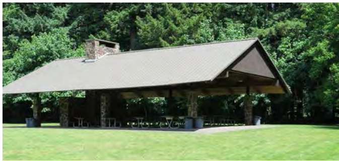
Existing River Shelter
