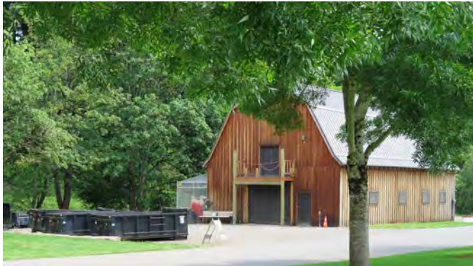
Future Picnic Shelter with Restroom
