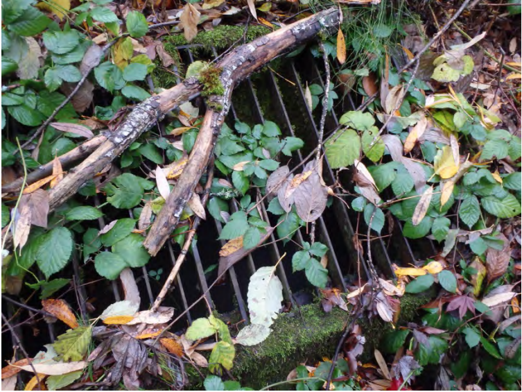
Photo 8 36-inch Outfall into Concrete Box
