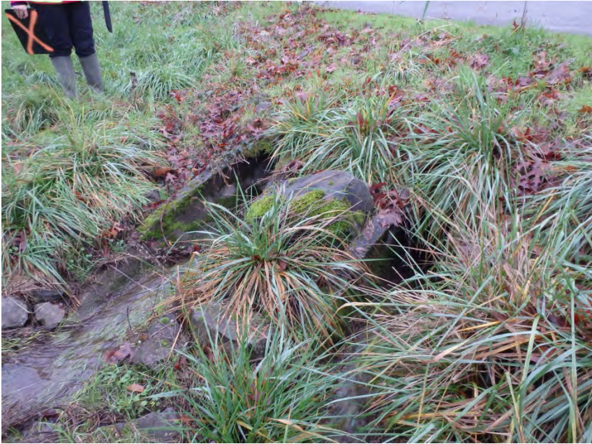
Photo 2 Upstream Ends of Culverts
