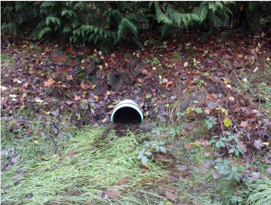
Photo 6 Partly submerged 18-inch CCP contributing culvert
