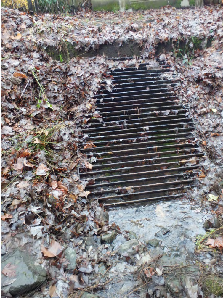
Photo 7 36-inch culvert under SW Willow Creek Drive
