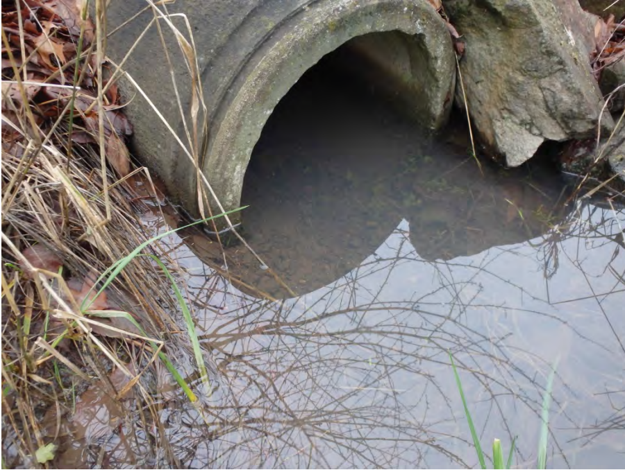
Photo 3 Downstream of culvert with gravel accumulation
