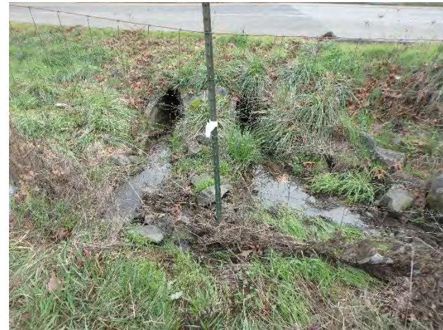
P28: Southern portion of Willow Creek and Culverts, looking south
