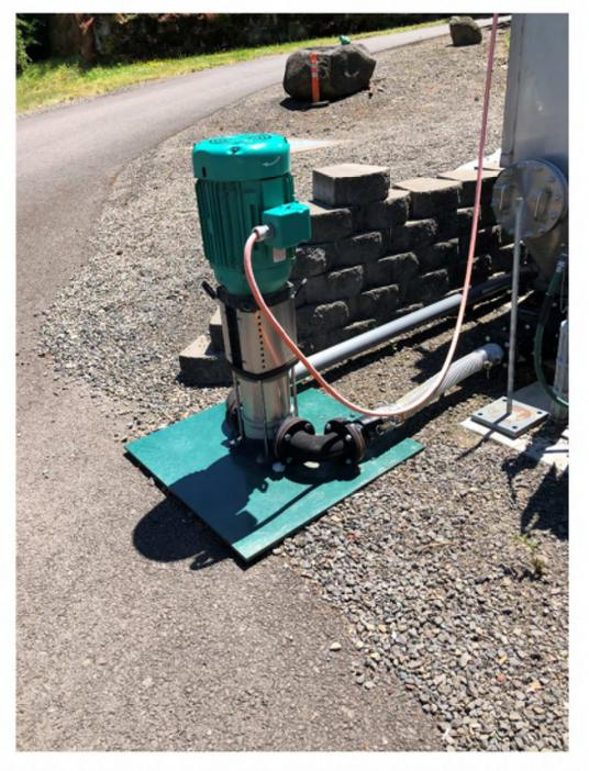
Recirculation pump is anchored to plate below, but there doesn't appear to be any support for equipment overturning.
