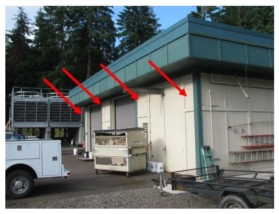
Figure 21 Workshop - East Elevation Shear Walls are Considered Narrow and Could Limit Strength
