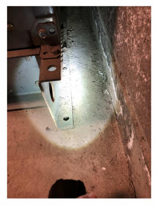
HVAC equipment is unanchored to structure along backside.
