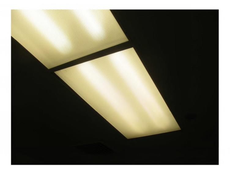
Lens covers within building lack safety devices. The covers currently can swing open without a latch.
