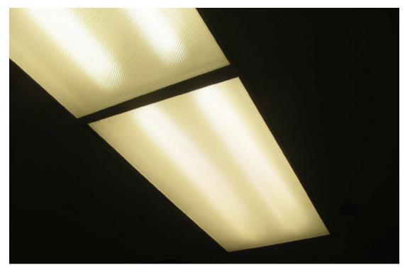
Figure 7 Operations Building - Lens Cover Lacks Safety Device
