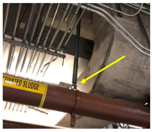
Figure 17 Process Gallery - RAS Piping Lacks Lateral Bracing Along Length at Compression Struts
