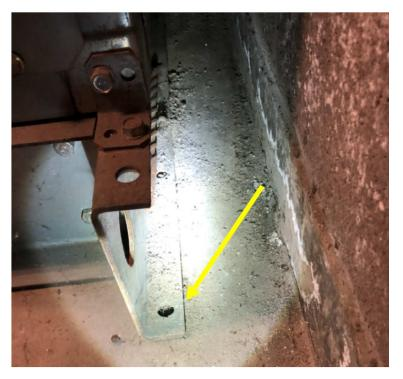
Figure 14Process Gallery - Air Handling Unit Lacking Anchorage
