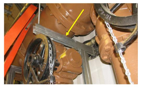
Figure 16 Process Gallery - Piping Lacks Connection Back to Supports Below
