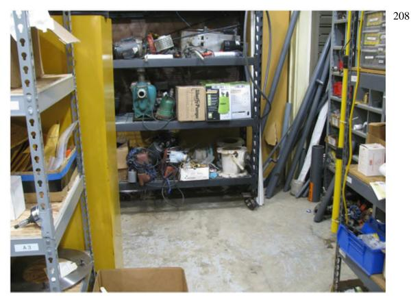
Storage rack shelves have wheels and free to move without restraint back to structure.
