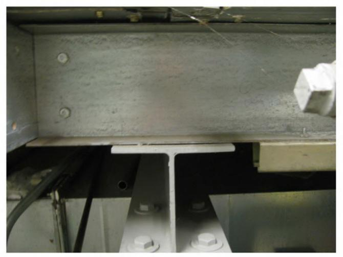
The HVAC equipment in Mechanical Room doesn't appear to be anchored to supporting structure framing below.
