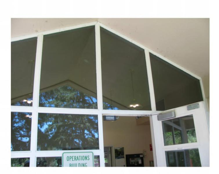
Exterior windows do not appear to meet requirements of heat laminated or have restraint to remain within frame if cracked.
