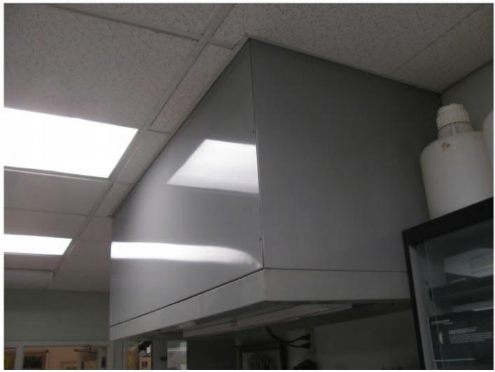
The laboratory hood equipment is assumed to be seismically unbraced.
