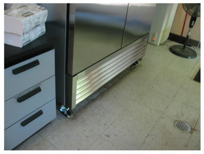
Refrigerator doesn't appear to be restrained laterally. There are rollers, but if set in lock position, there is potential for overturning.
