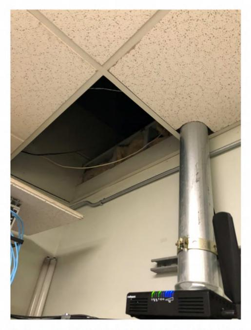
Ceiling supported off wall. There is no gap between ceiling channel edge and wall.
