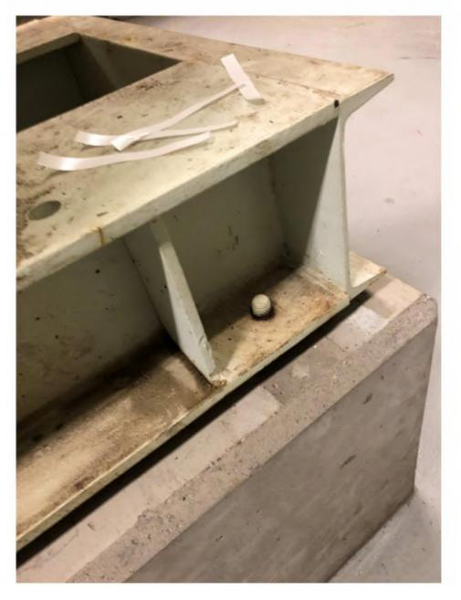
Aeration blower pump lacks anchorage to structure. Nuts are missing or backing off from threaded rods.
