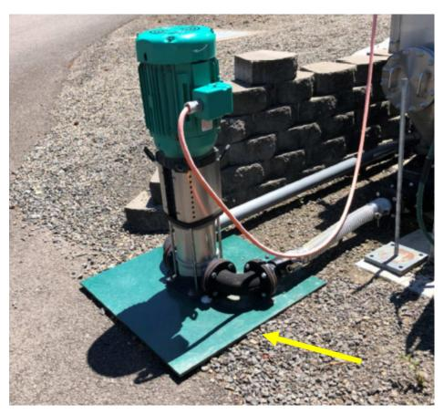
Figure 30 Disk Filters - Recirculation Pump Lacking Resistance to Overturning
