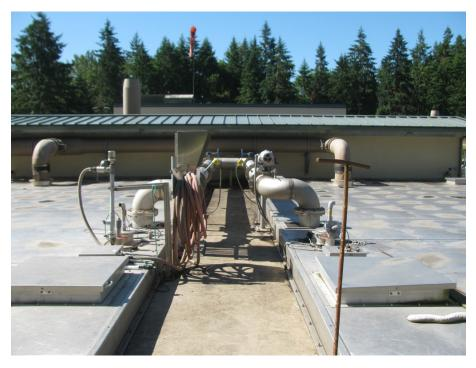
Figure 26 Stabilization Basin - Walkway with Piping and Support
