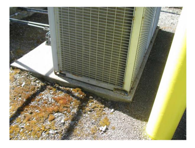
ACCU units lack anchorage to structural pad near Aeration Basins.
