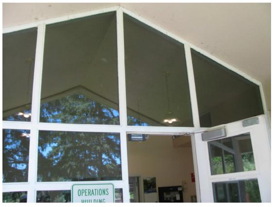
Figure 8 Operations Building - Window Above Entrance Appears to Lack Special Treatment to Limit Damage
