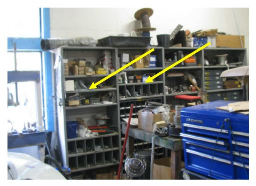
Figure 23 Workshop - Storage Shelves on South Wall Missing Anchorage
