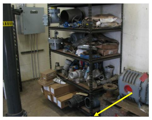
Figure 29 Headworks Building - Shelving Lacks Anchorage to Structure
