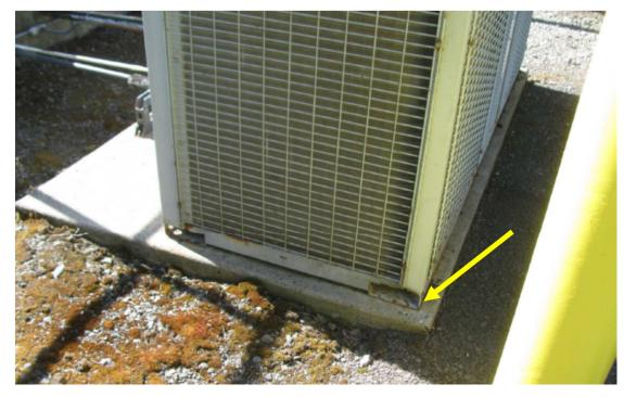
Figure 31 Aeration Basins Canopy - ACCU Units Lacking Anchorage To Concrete Pad
