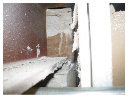
Figure 9 Operations Building - Collector Beam Connection to CMU Wall
