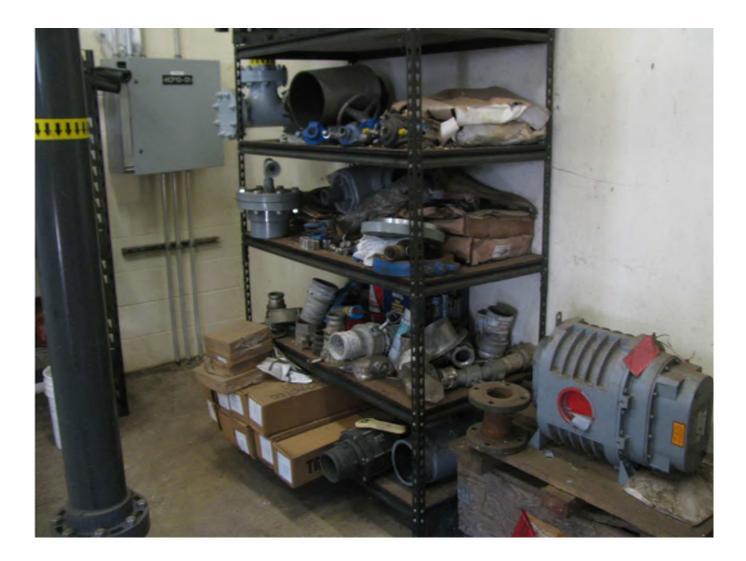
Storage racks within the Headworks building appear to be unanchored to structure.
