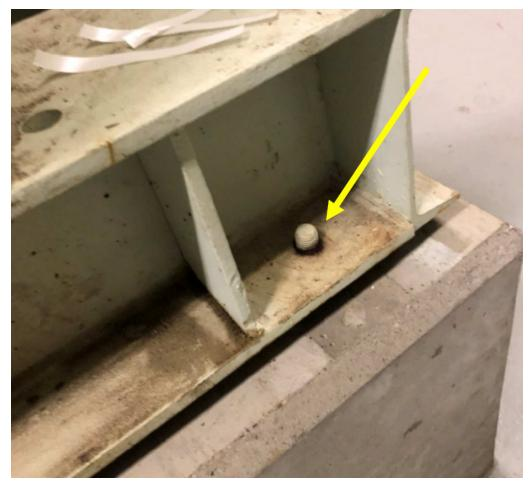
Figure 15 Process Gallery - Blower Equipment with Missing Nuts
