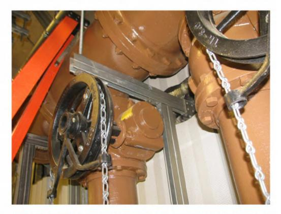
Piping lacks restraint to unistrut support. Pipe shown is sitting on unistrut.
