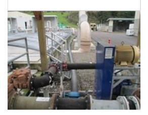
These vertical, submersed progressing cavity pumps were undersized (50 GPM). Are currently unused, replaced with Vogelsang rotary lobe pumps.
