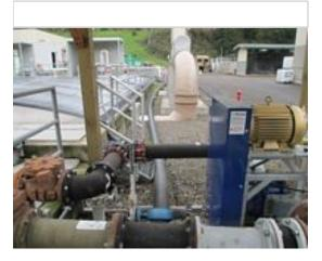
These vertical, submersed progressing cavity pumps were undersized (50 GPM). Are currently unused, replaced with Vogelsang rotary lobe pumps.
