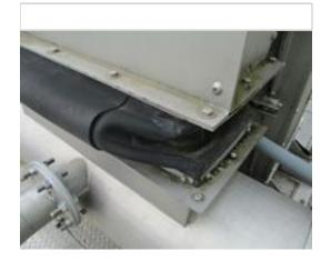
Deterioration of rubber between screen and screening trough
