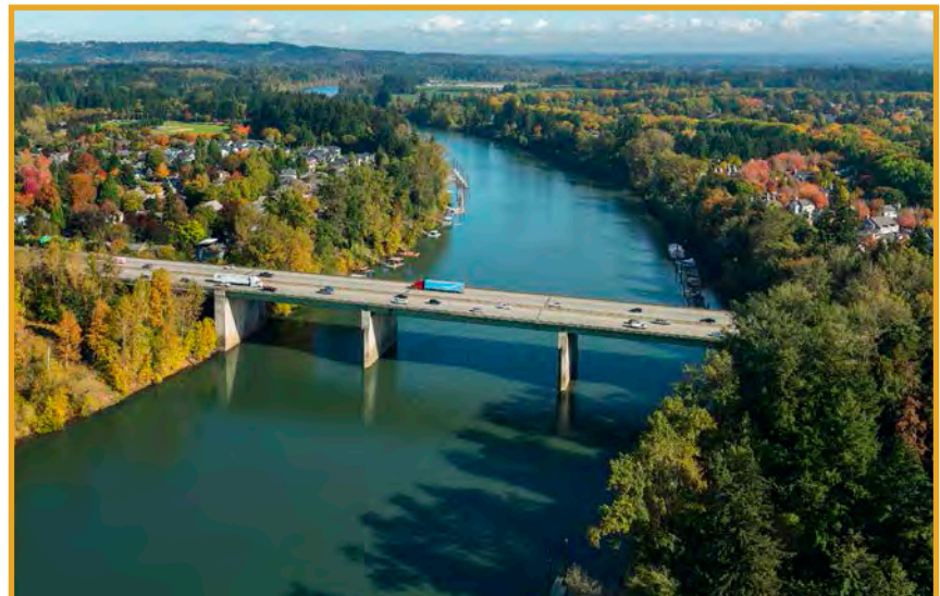
Above: The I-5 Boone Bridge.
