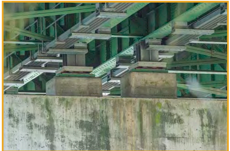
Above: Existing railing and pier supports of the Boone Bridge.
