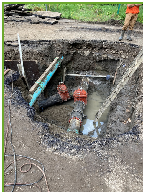
Temporary diversion of wastewater
