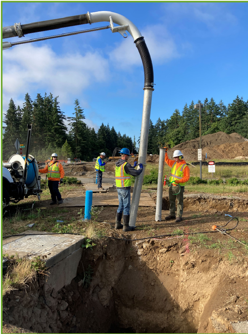
Potholing to find the water line
