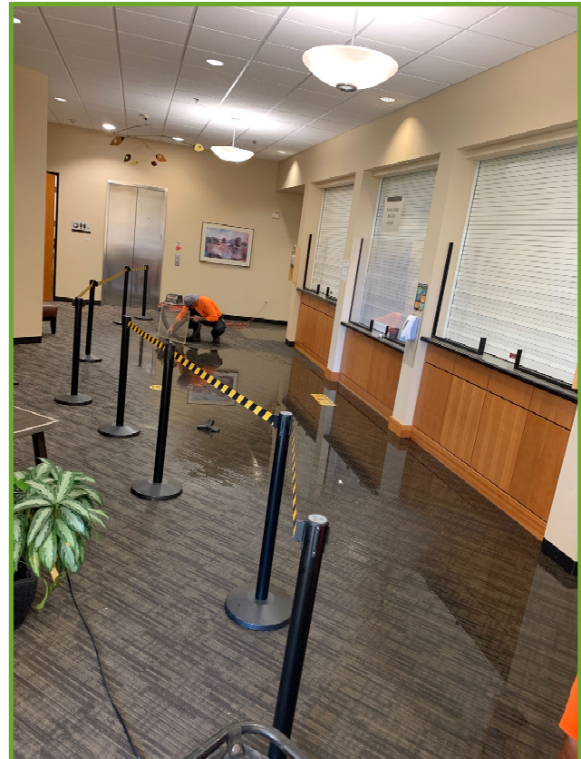
Cordoned off work site
