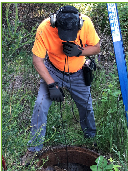
Listening for a leak
