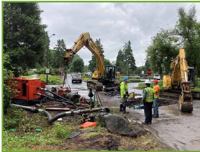
Excavating the old force main pipe
