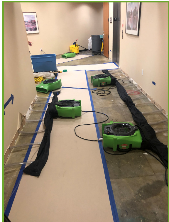
Drying the lobby —the elevator stayed dry!
