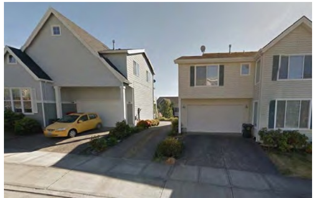
Homogeneous homes, without adequate detailing and landscaping, detract from the attractiveness of the neighborhood.
