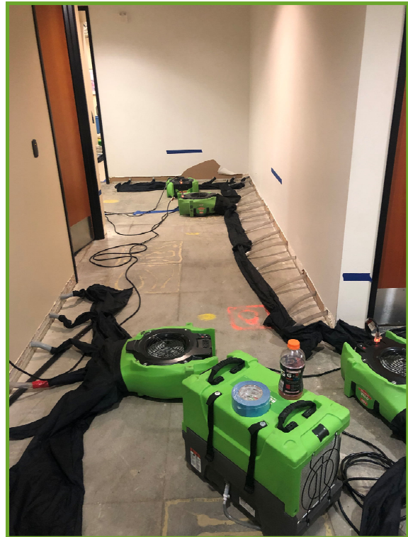
Drying the hallways outside the restroom
