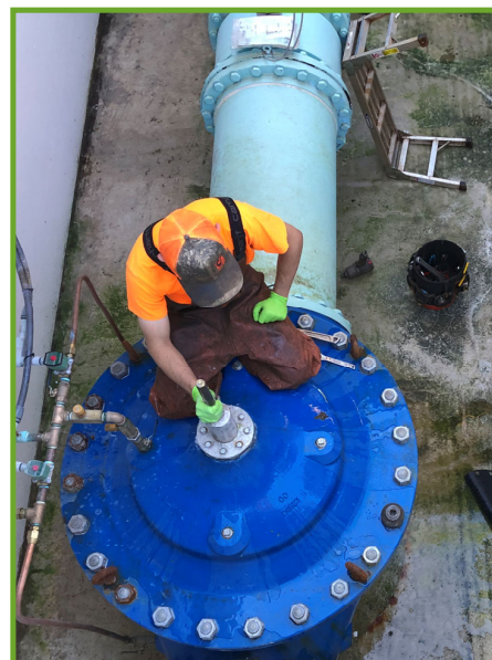
Control valve maintenance
