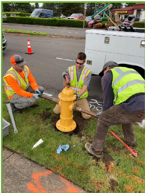
Setting new hydrant
