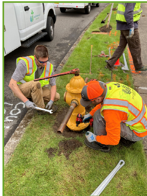
Securing the new hydrant
