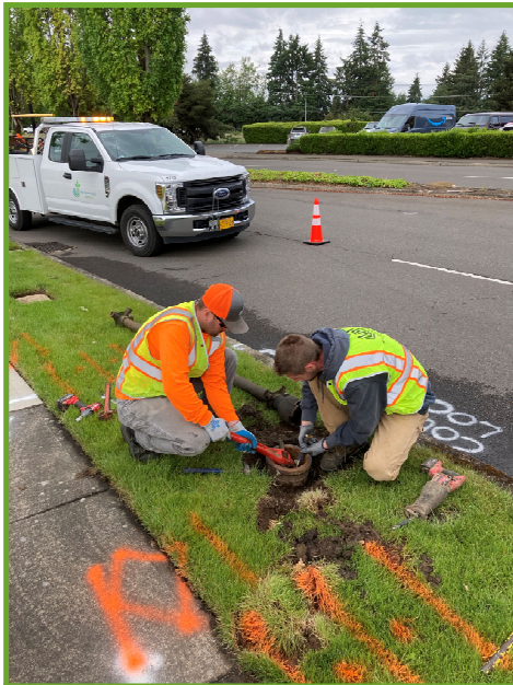
Removing inner stem
