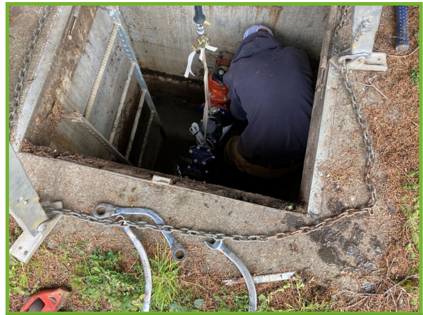
Sam performs a meter replacement
