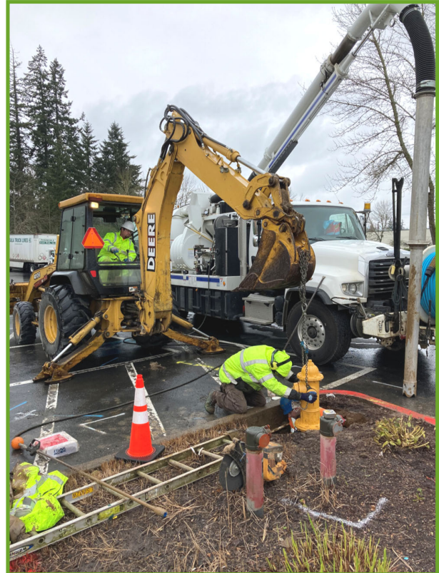
Installing a new hydrant
