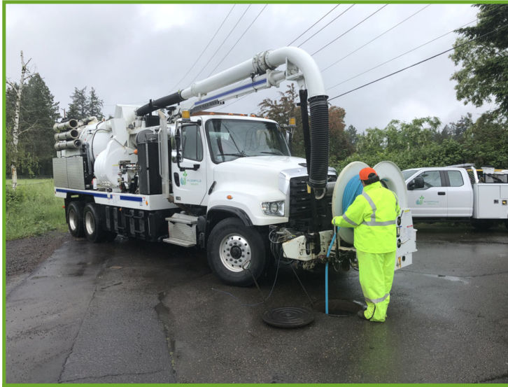
Flushing the sewer line
