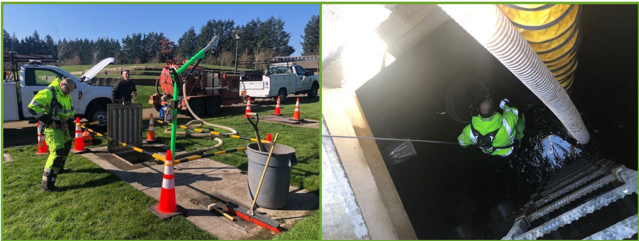
Preparation and entering an underground confined space
