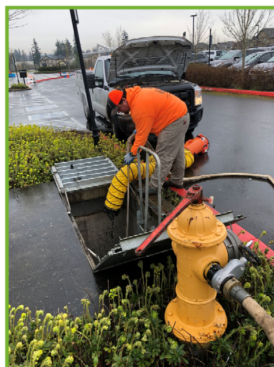
Chad cleaning vault
