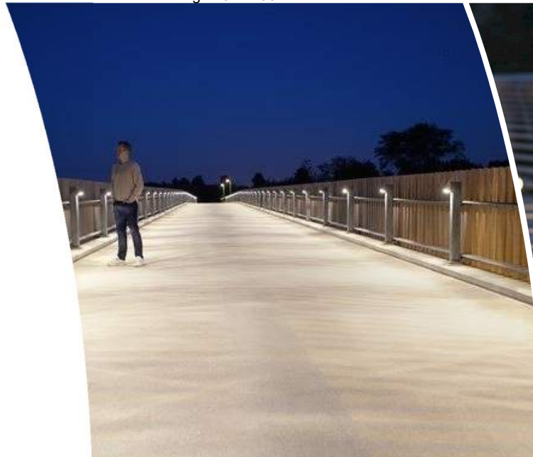
Intermittent Handrail Lighting
