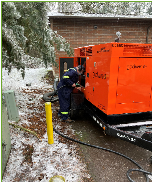
Refueling the portable pump
