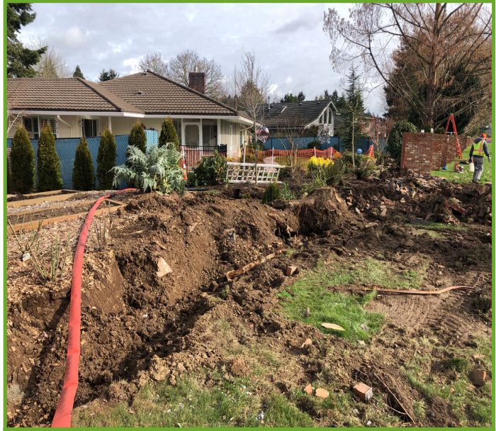
Miley Road Pipe Repair Project
