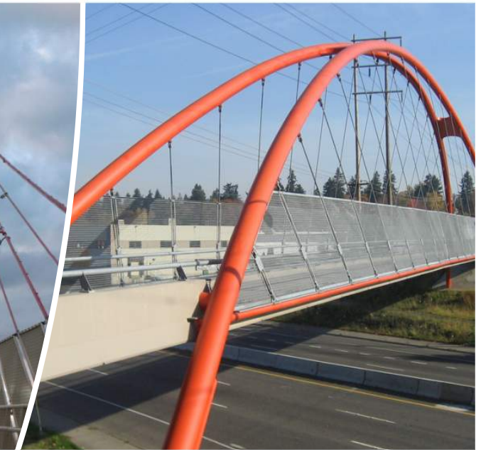
Springwater Trail Bridge
