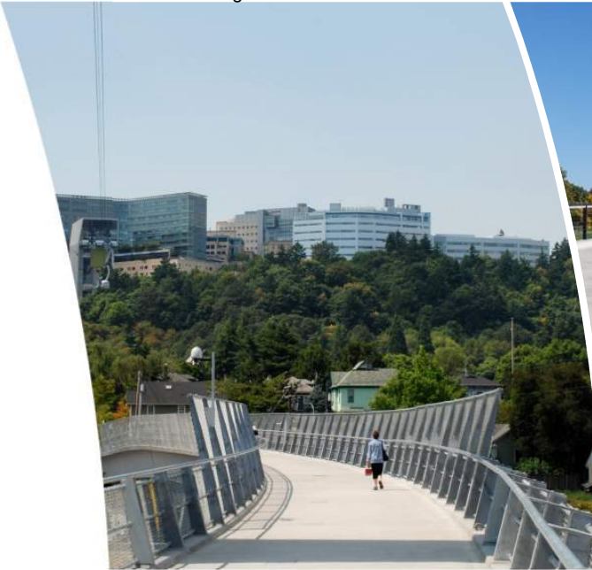
Gibbs Street Bridge
