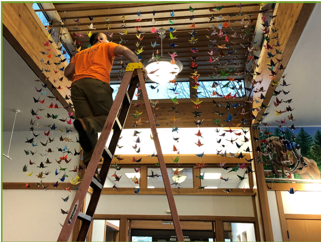
Starting the installation of Soaring Spirits
