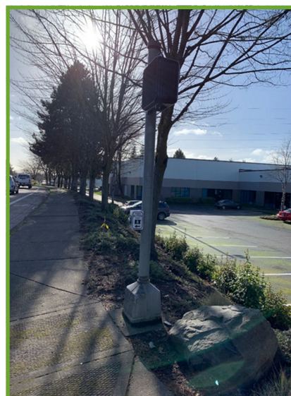
New crosswalk signal
