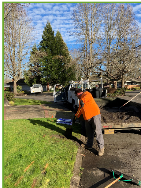
Backfilling the pothole
