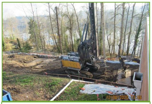
Drill rig for deep soil mixing which will provide seismic stability of the Willamette River bank.
