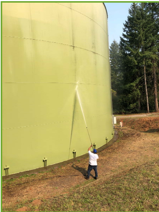
Pressure washing the sides
