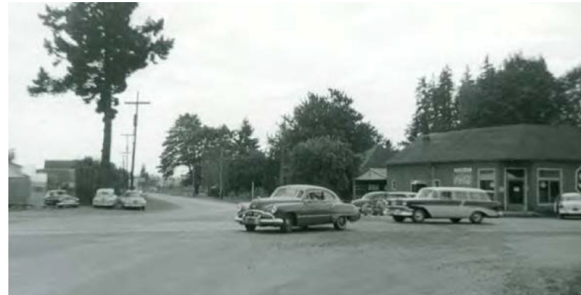
Intersection of Wilsonville Road and Boones Ferry Road, circa 1950. Credit: Wilsonville-Boones Ferry Historical Society.
