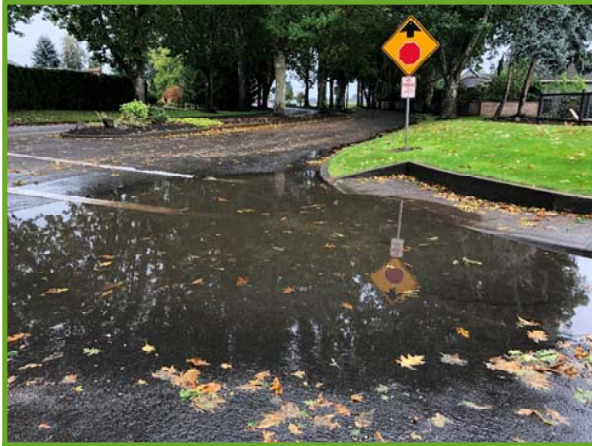
Standing water at crosswalk
