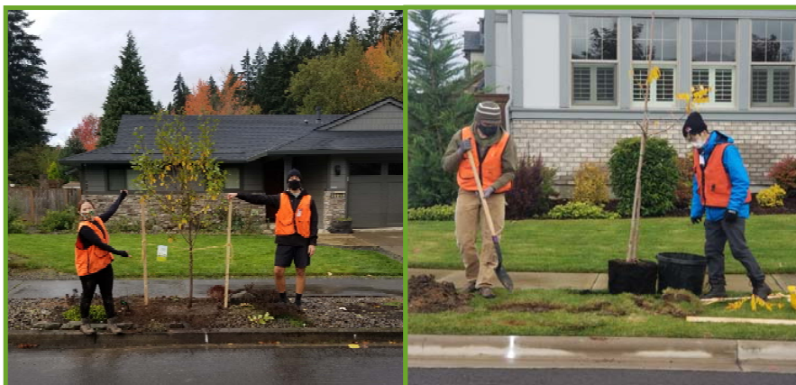
Friends of Trees staff and trained volunteers installing street trees around the City
