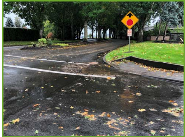
After clearing curb inlet
