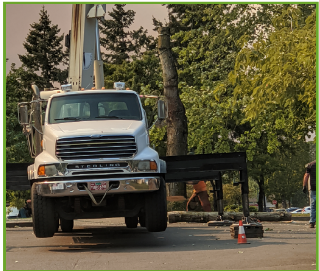
Tree removal at Public Works
