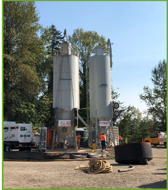
Mixing plant to create slurry for the deep soil mixing along the Willamette River bank
