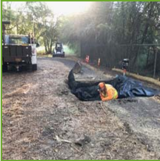
Digging by hand
