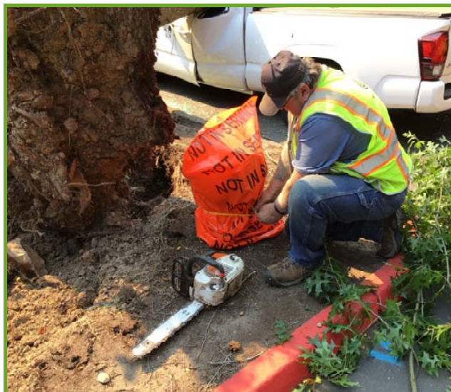
Water Technician Jerry Anderson bagging hydrant
