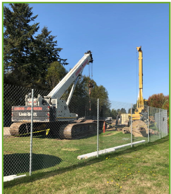
Yet another crane and drill rig for the RWF_1.0 work
