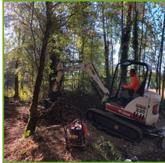
Using an excavator to move dirt
