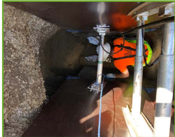
Working in the trench
