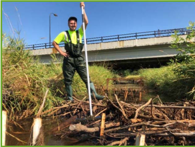
BEFORE— built up debris pile
