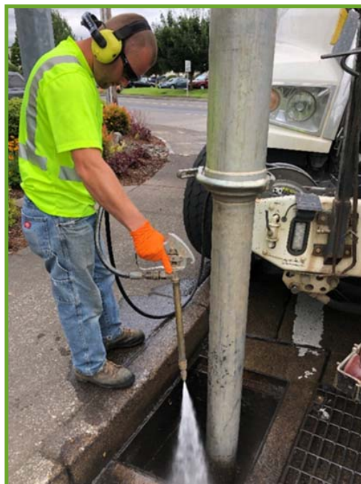
Cleaning catch basin
