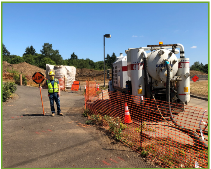
Controlling pedestrian traffic during construction
