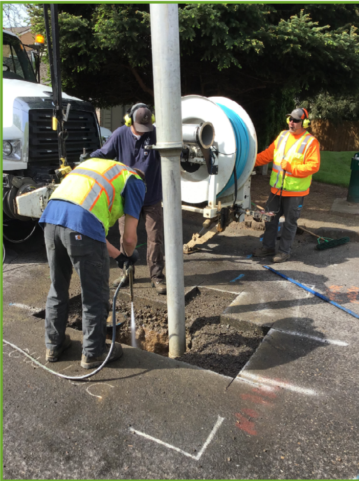
Using the vacuum truck to excavate trench
