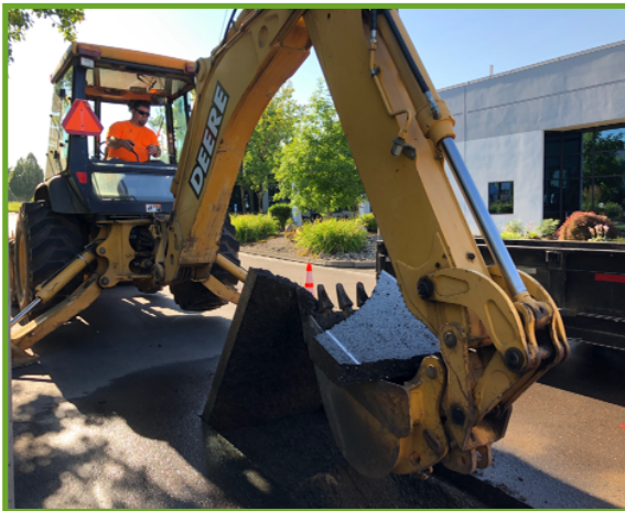
Removing Asphalt
