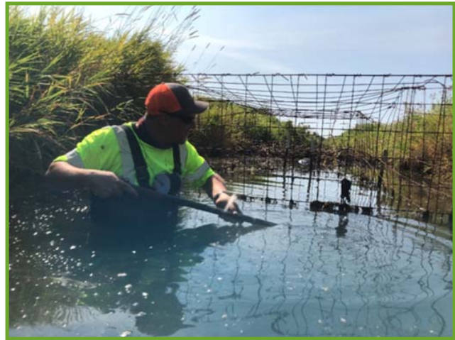
AFTER—water flowing again
