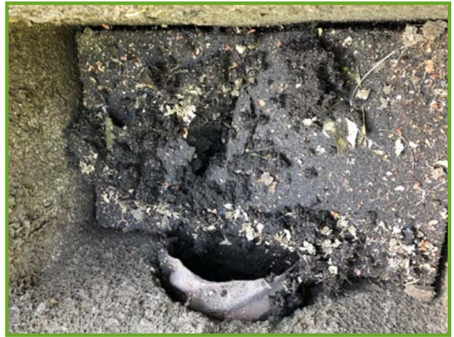
During—can start to see pipe
