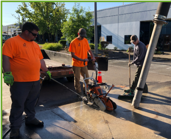
Cutting Concrete
