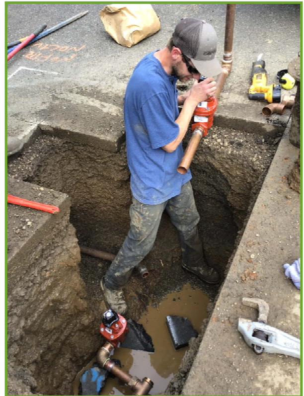
Installation of blow off valve
